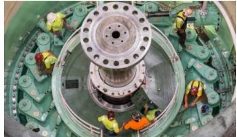
Chief Joseph Dam Powerhouse
