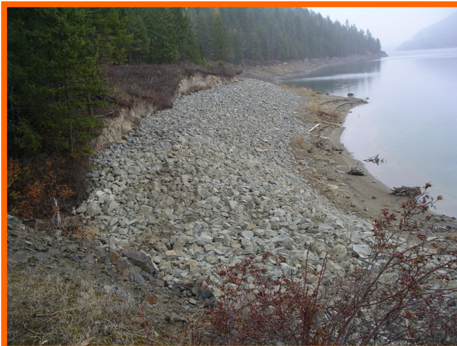
Stabilization of the Barron Creek Site
