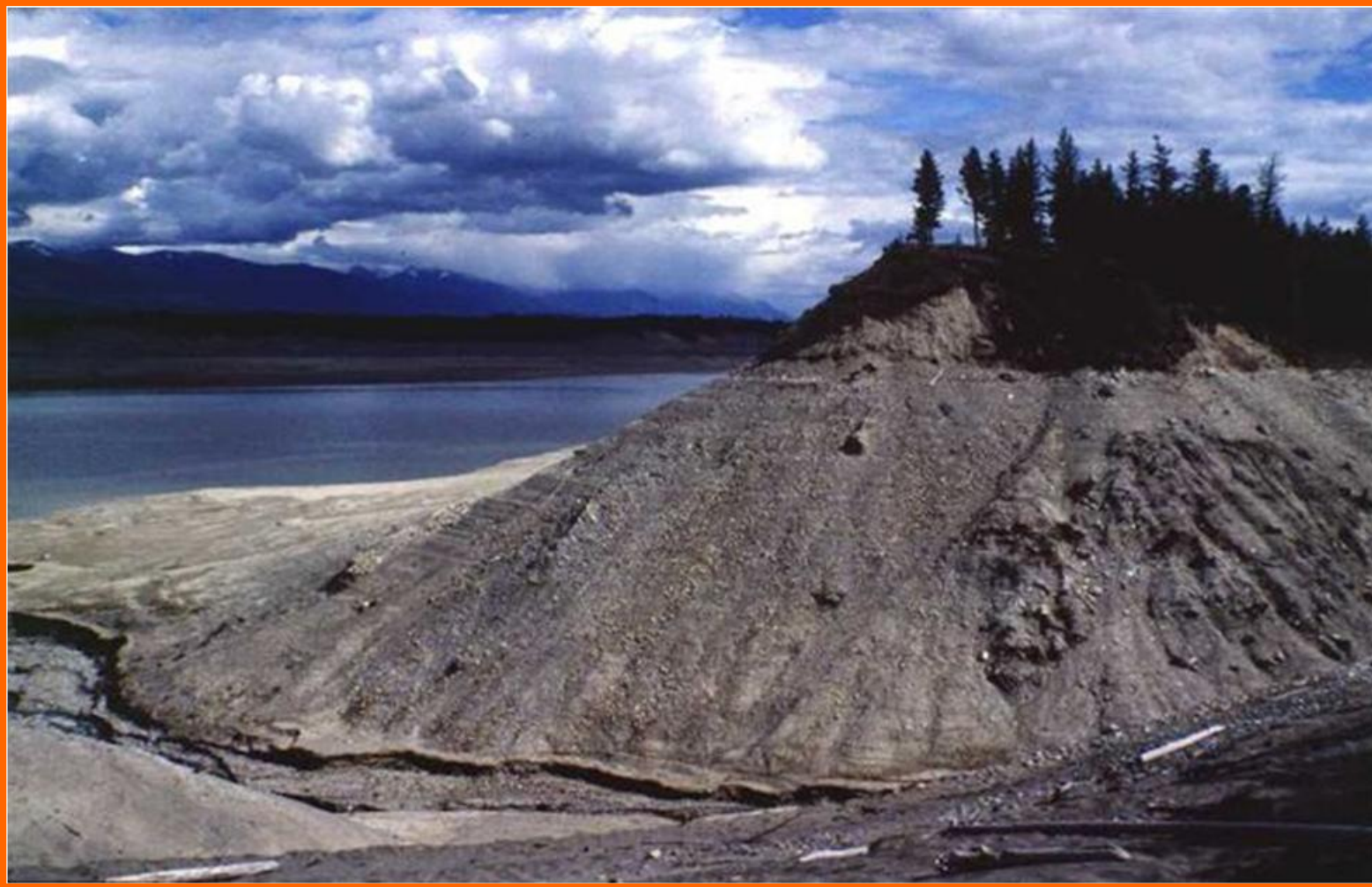
Erosion at the Libby Dam Project
