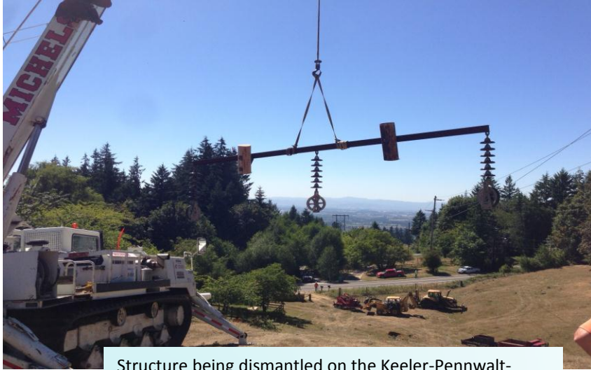
Structure being dismantled on the Keeler-Pennwalt-115kV line at the southern Boundary of Forest Park. Part of retiring two de-energized 115kV lines running from Keeler Substation through Forest Park.
