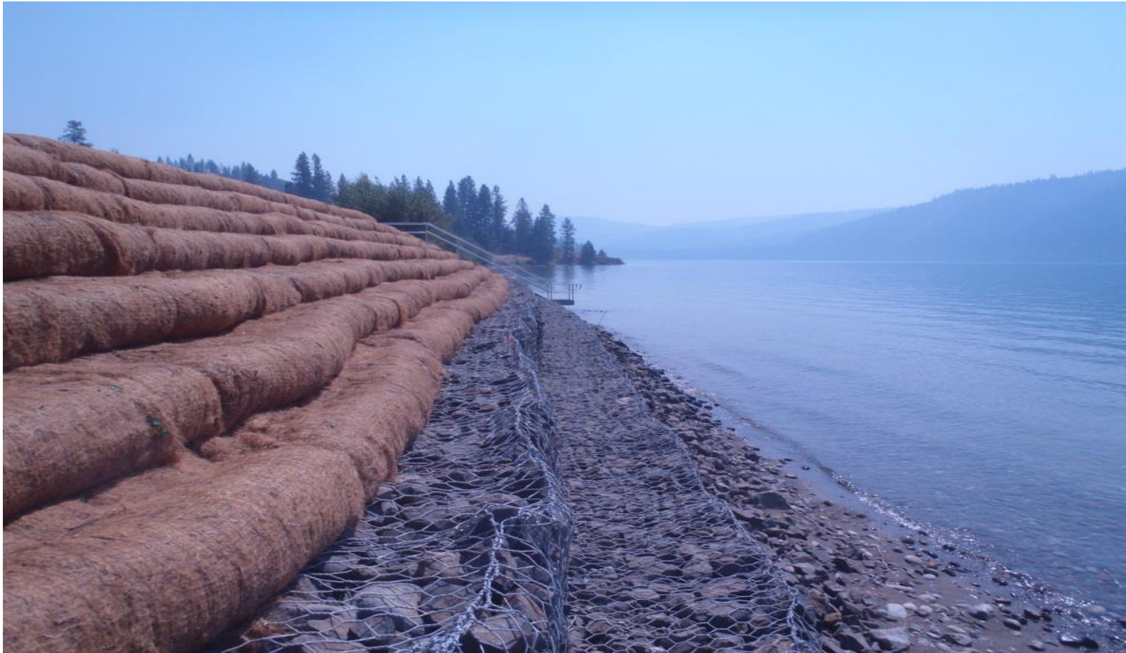
Stabilization of reservoir bank to reduce erosion of artifacts from an archaeological site Grand Coulee project
