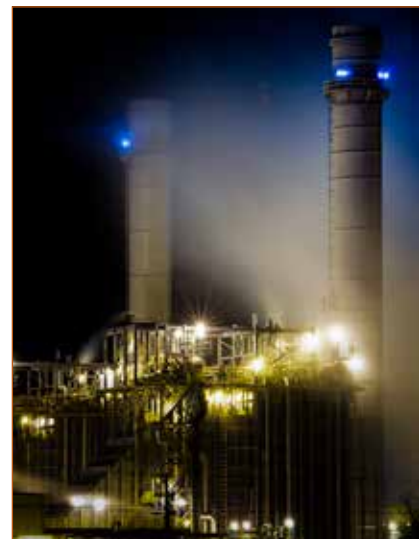
Natural gas power plants emit half the amount of carbon dioxide into the atmosphere as coal-fired plants. Recent advances in gas production technology have led to bountiful natural gas and a technology revolution in energy production. But due to lower costs, natural gas would also replace some low-carbon energy, such as renewables or nuclear energy. Photo courtesy of Scott_Butner@charter.net.
