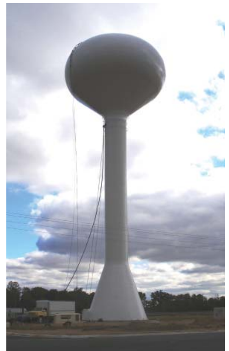
Sarah Hudson, Indiana DWSRF Elevated storage tank in Greensburg, Indiana.
