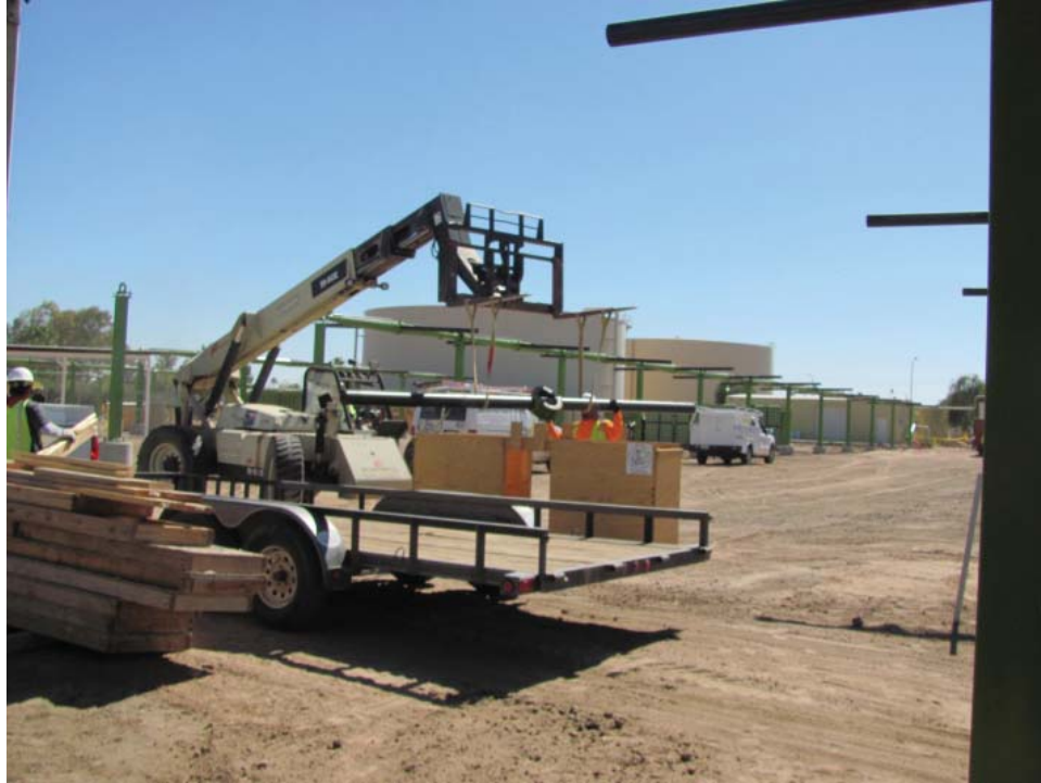
Water Infrastructure Finance Authority of Arizona
