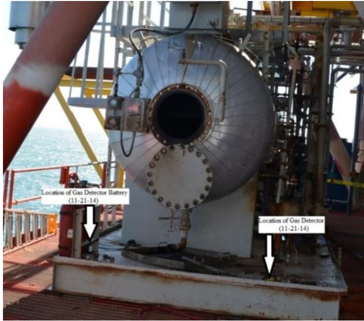
Figure 30 - Gas Detector Unit and Battery Locations (November 21, 2014)
