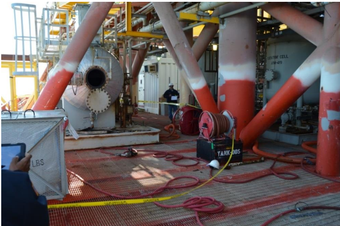
Figure 11 - Production Deck and Heater Treater (November 21, 2014)
