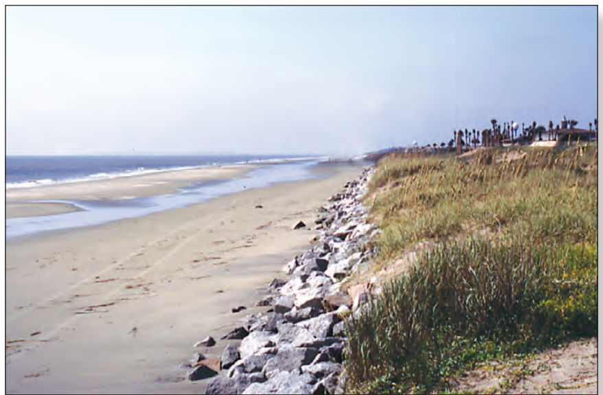
Figure 38. Shoreline armoring and stabilization along this beach in North Carolina was designed to protect coastal dunes and development.
