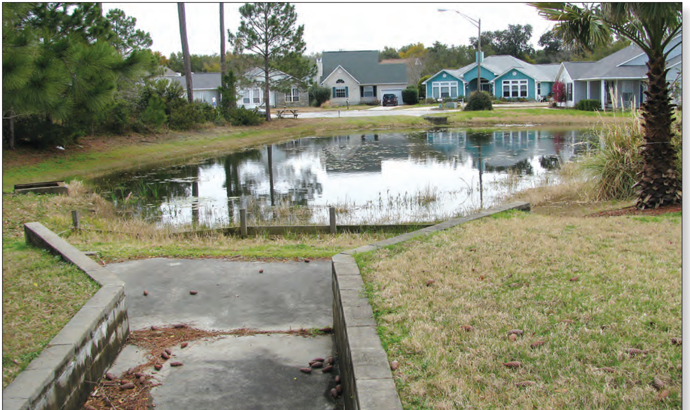
Figure 54. A created pond in an urban subdivision has been used to drain an adjacent vegetated wetland and serves as a retention basin to compensate for the increase in impervious surface from the development.
