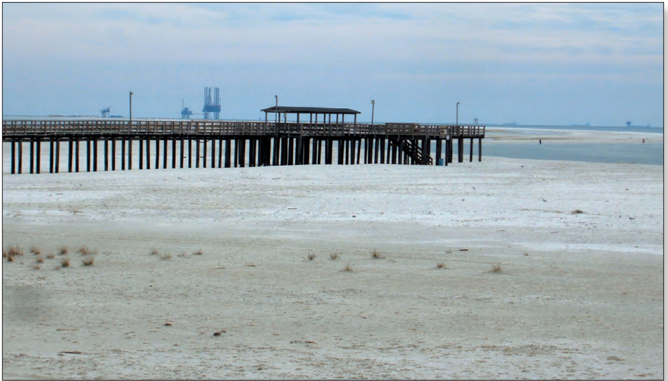
Figure 34. The fishing pier on Dauphin Island, Alabama, no longer reaches the water line as coastal sediments have been deposited along this shore (2010).
