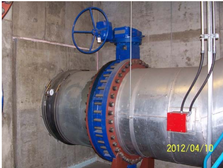
Figure 3.6. Location of Tracer Injection in Building 160. The smoke detector (red box) was removed and the existing duct penetration was used for the injection port.
