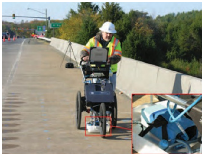
Figure 2.21. Depiction of GPR Testing on Transportation Infrastructure (TRB 2013)
