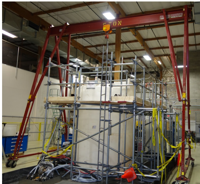
Figure A.3. Scaffolding and Gantry (before two additional cranes/hoist installed).
