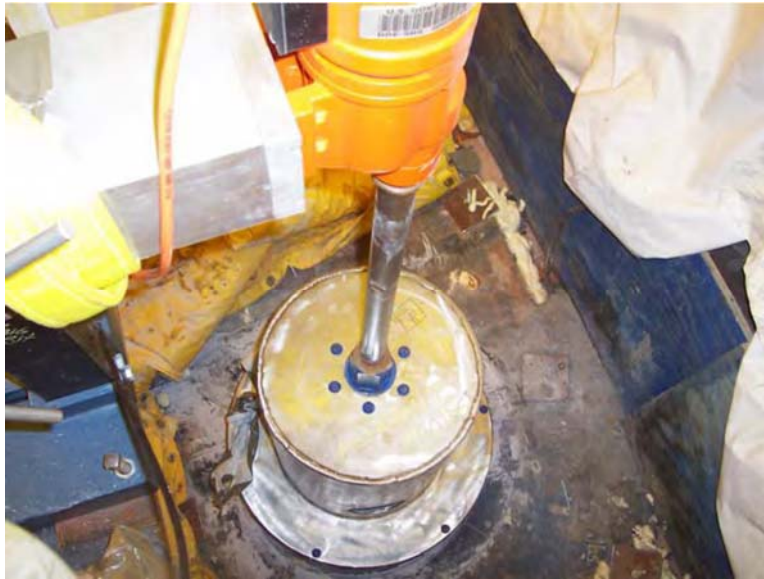
Figure 4-3. Core Drilling of New Mechanical Cleaning Riser in Tank 18
