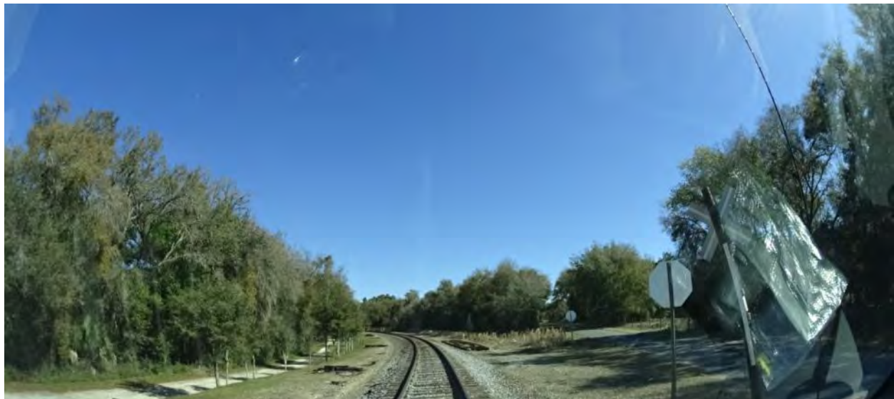
Figure 2-163. Florida Northern Railroad near Dunnellon, Florida (2015)
