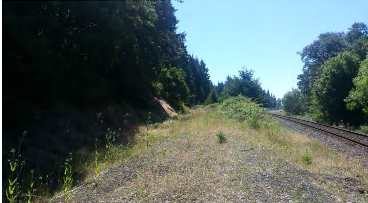
Figure 2-104. Former Trojan Rail Spur Railbed (2013)
