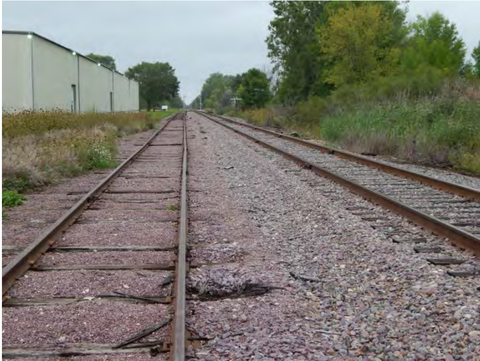
Figure 2-210. Potential Bellevue Transload Location (Looking North) (2014)
