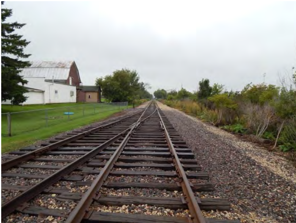
Figure 2-204. Potential Luxemburg Transload Location Further Down Track (Looking West) (2014)
