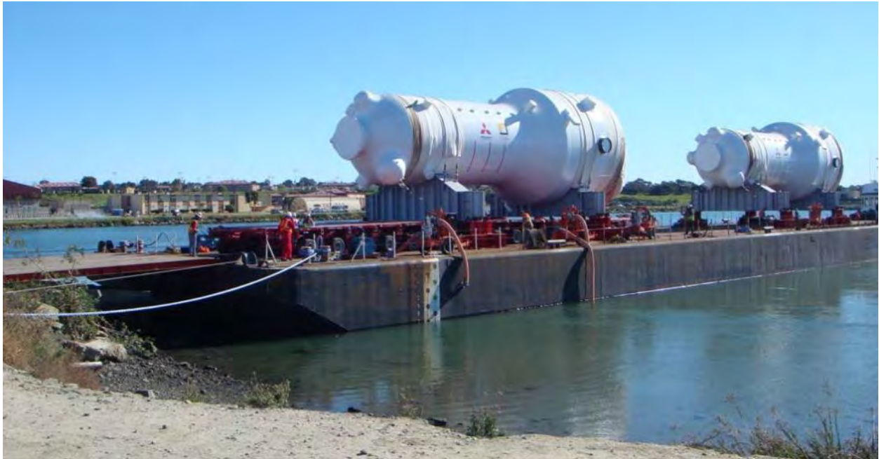
Photo courtesy of California Public Utilities Commission
