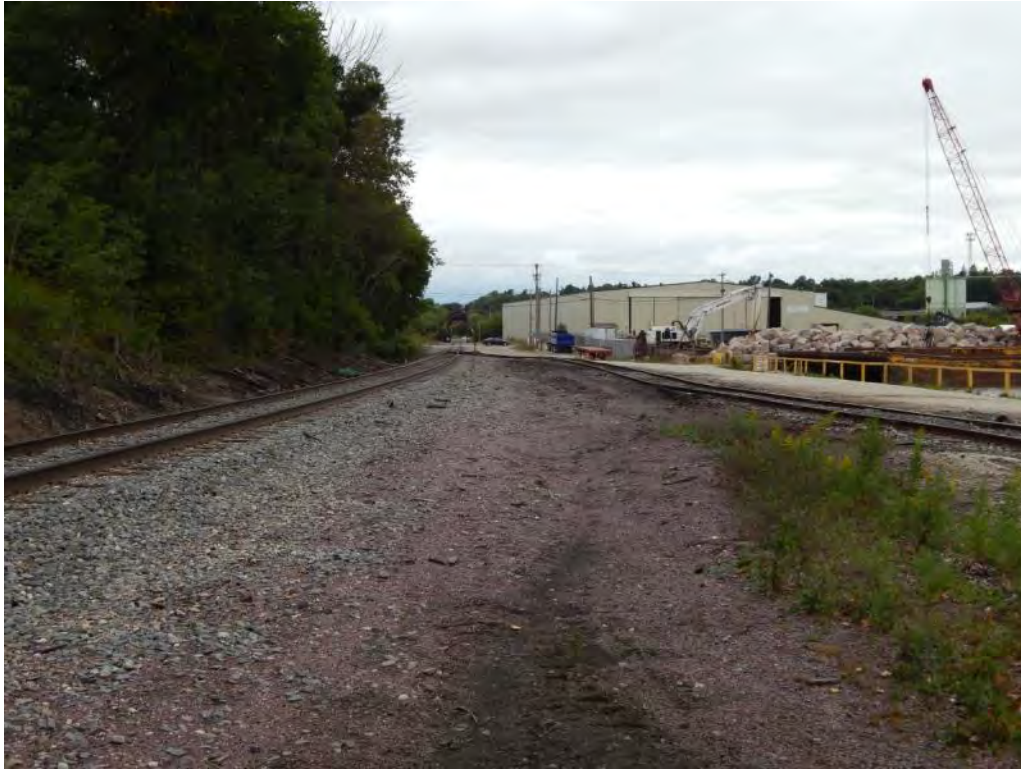
Figure 2-236. Potential Manitowoc Transload Location (Looking Northwest) (2014)
