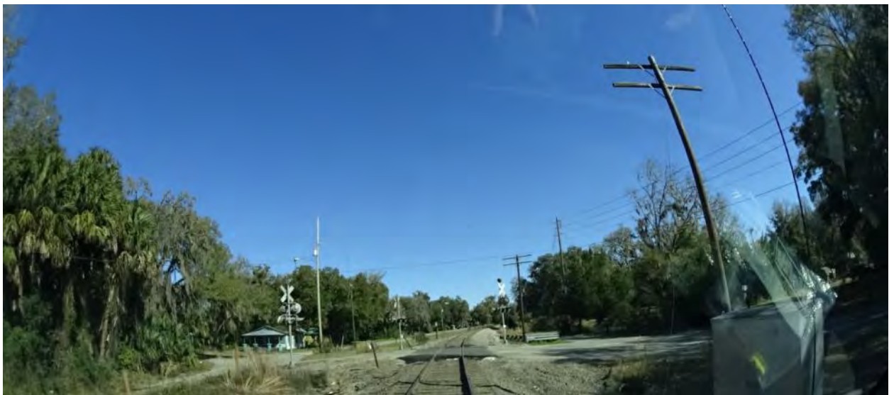
Figure 2-165. Florida Northern Railroad Grade Crossing (2015)
