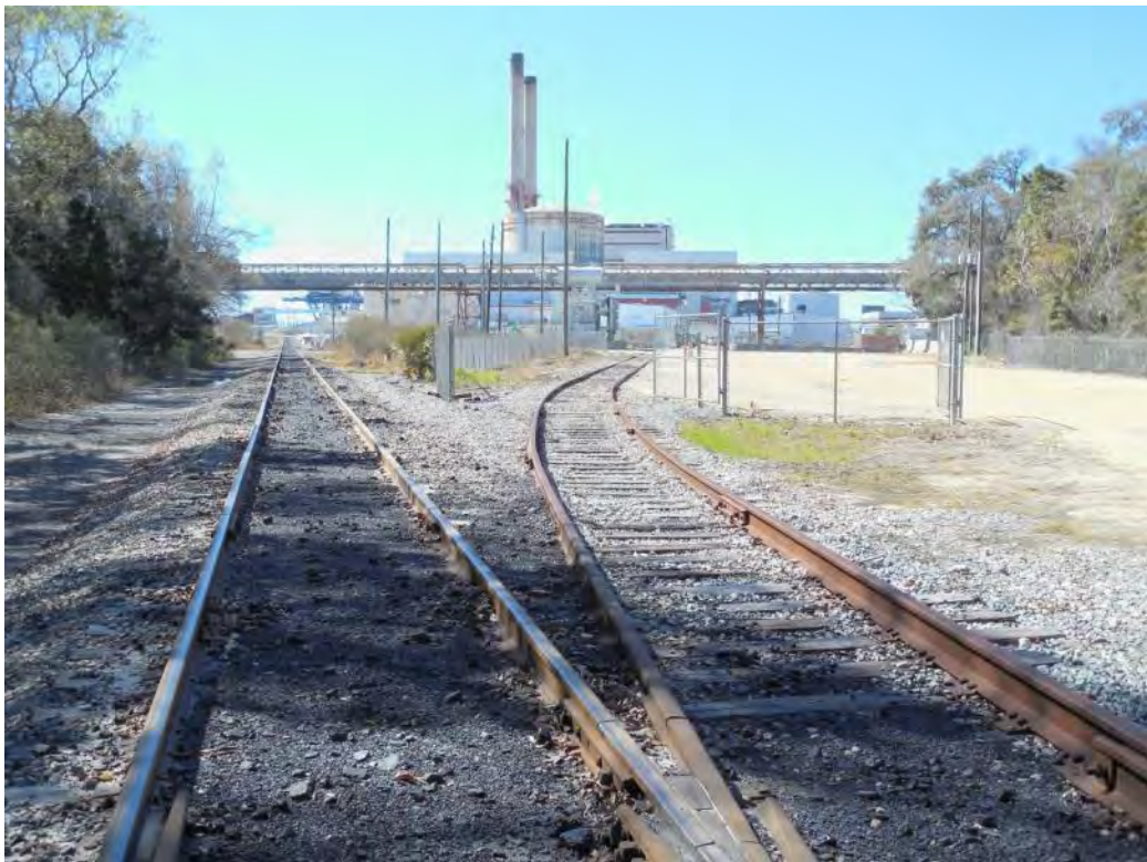
Figure 2-152. Junction of Onsite Industrial Spur (Left) and Nuclear Spur (Right) (2015)
