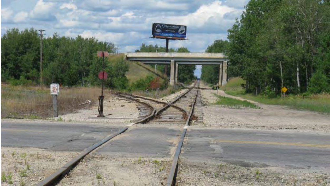
Figure 2-73. Condition of Rail Crossing Used for Big Rock Point Reactor Pressure Vessel Transload (Looking North) (2013)
