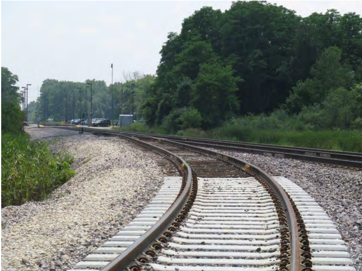
Figure 2-142. Junction of Zion On-site Rail Spur with Union Pacific Railroad Showing Concrete Rail Ties (2013)
