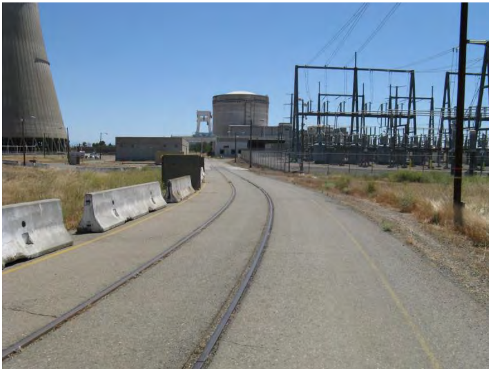
Figure 2-88. On-site Rail Spur Running into Rancho Seco Site (2013)
