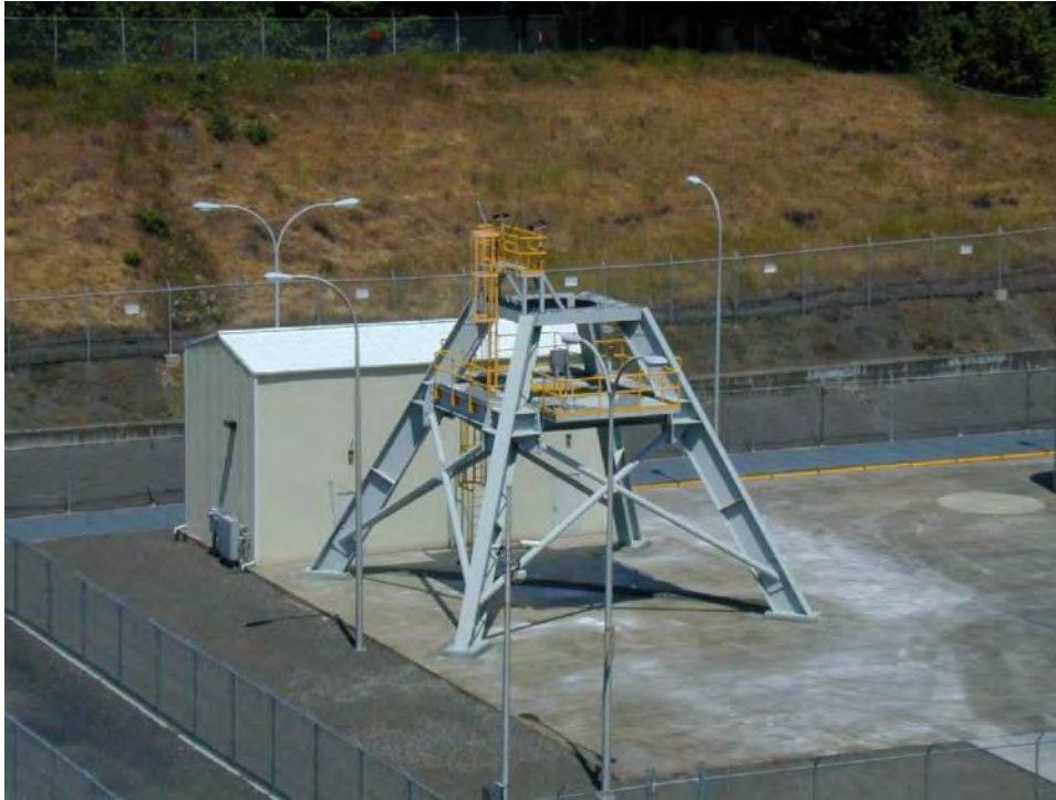
Photo courtesy of Trojan
