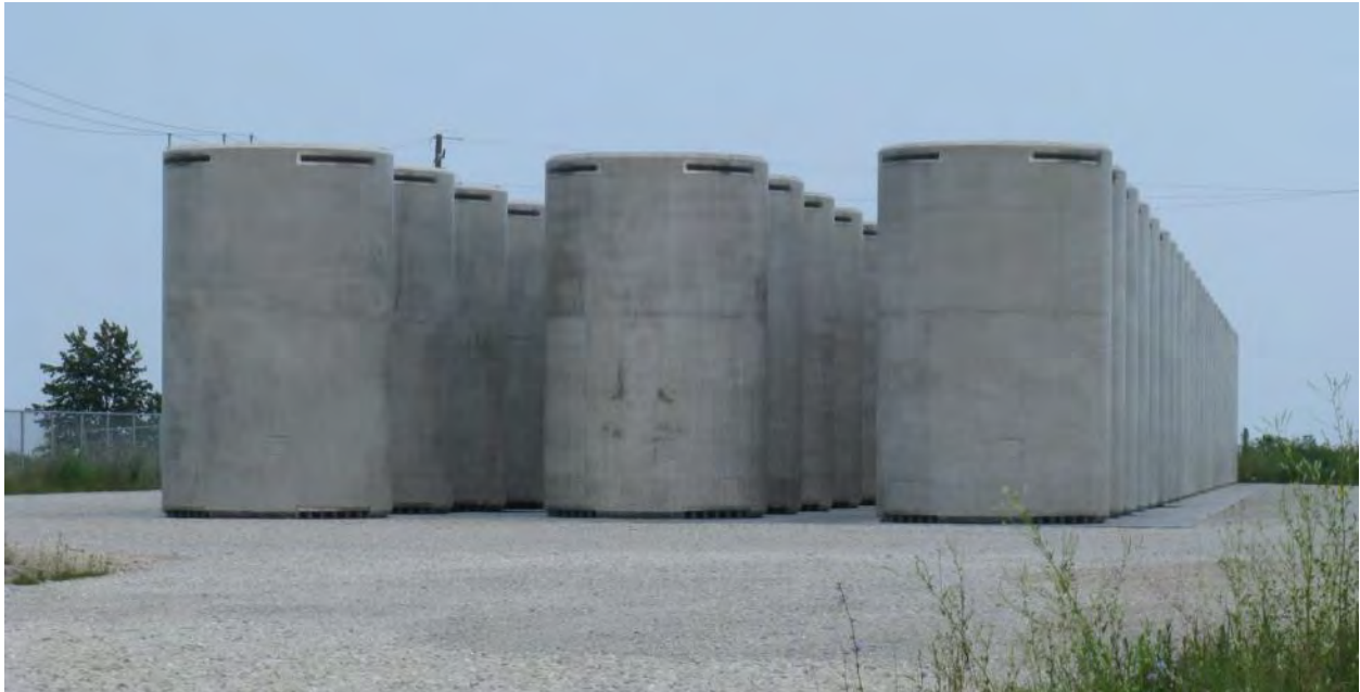
Figure 2-134. Vertical Concrete Storage Casks Staged at Zion (2013)
