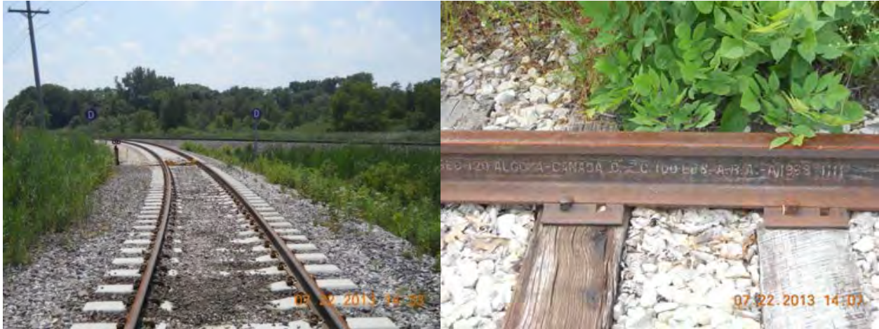
Figure B-17. Rebuilt Lead from the Zion Site to the Union Pacific Mainline (2013)
