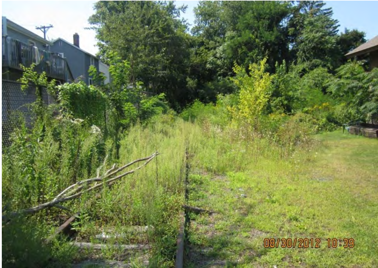
Figure 2-37. Conditions at the End of the Portland Rail Spur (2012)
