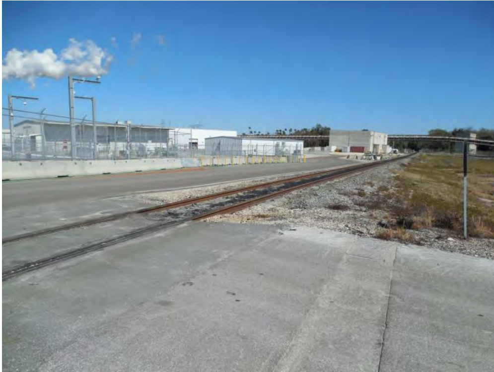
Figure 2-153. Onsite Industrial Rail Spur in Front of the Future Independent Spent Fuel Storage Installation Site (Facing East) (2015)
