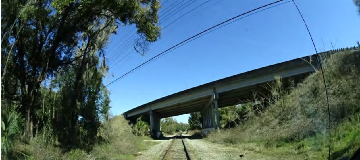
Figure 2-164. Highway Bridge over Florida Northern Railroad (2015)
