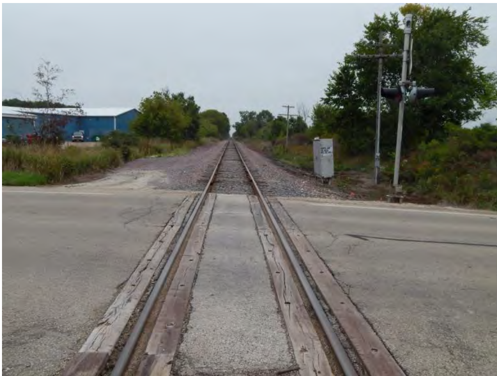
Figure 2-219. Potential Denmark Transload Location (Looking North) (2014)
