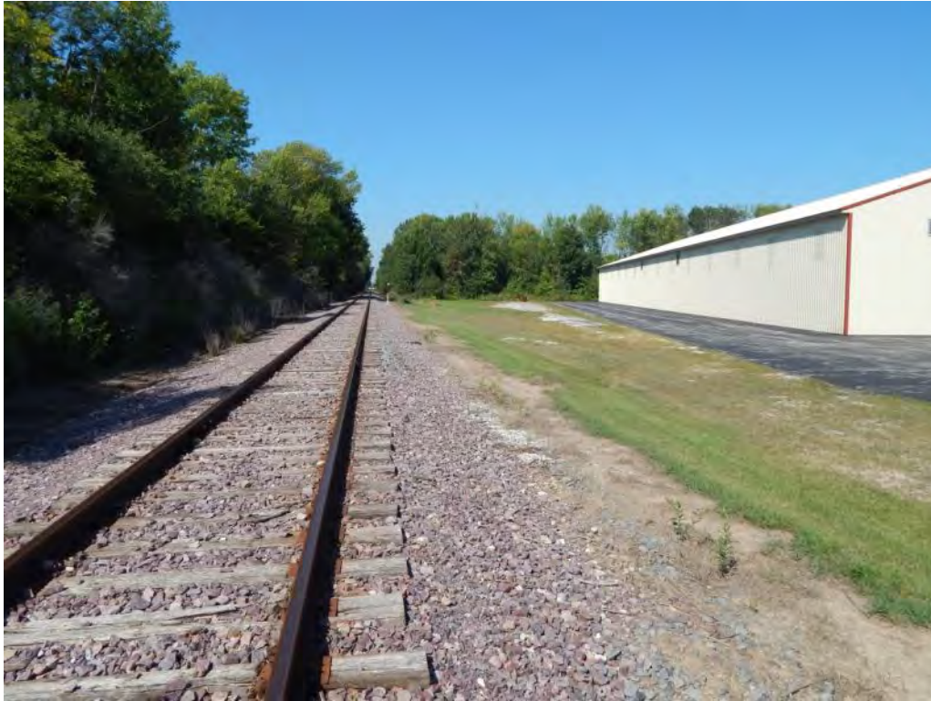
Figure 2-224. Potential Rockwood Spur at WI-310 Transload Location (Looking North) (2014)
