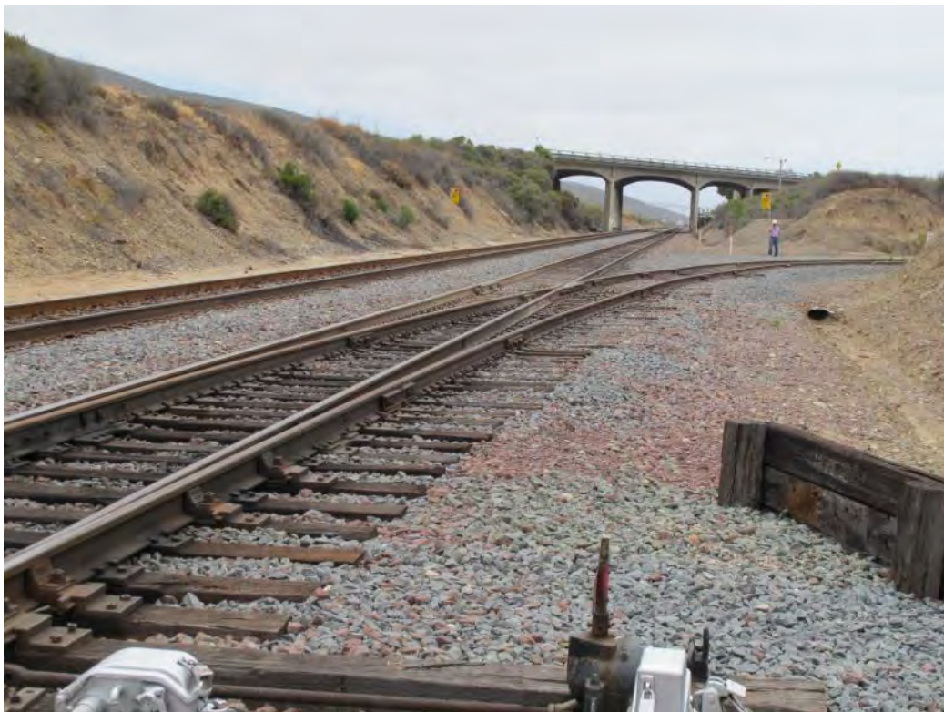
Figure 2-281. Mainline at San Onofre Site (Looking South) (2015)
