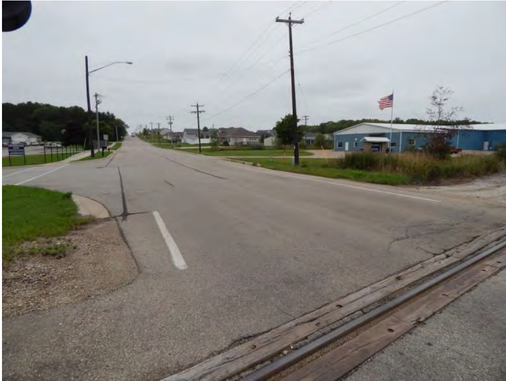
Figure 2-220. Potential Denmark Transload Location (Looking West) (2014)
