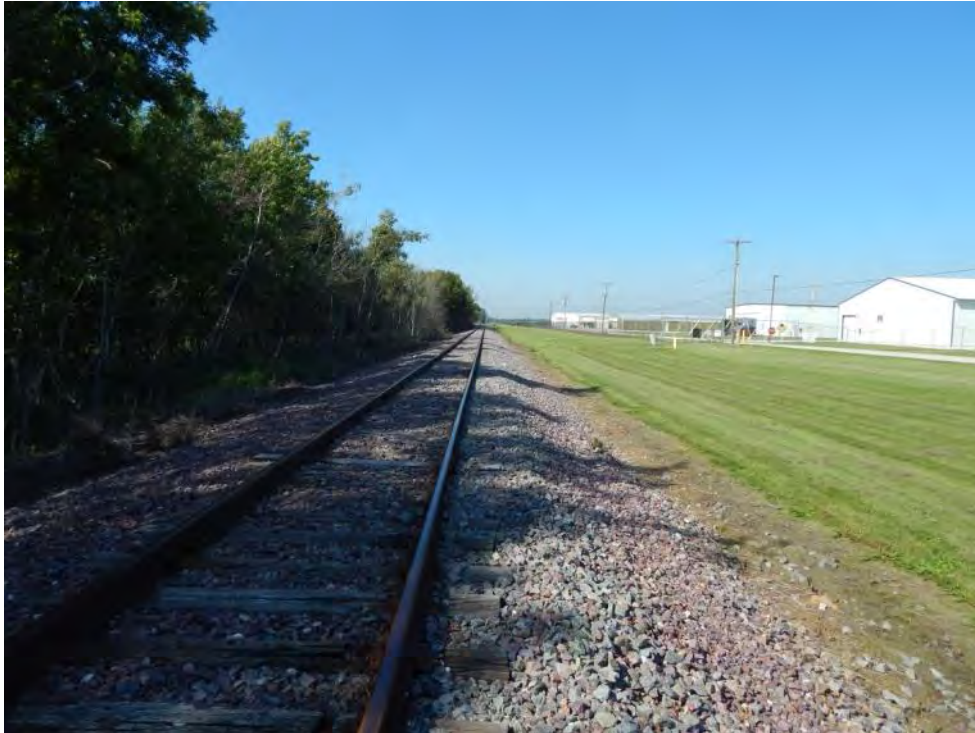
Figure 2-231. Potential Rockwood Spur at the Manitowoc Airport Transload Location (Looking North) (2014)
