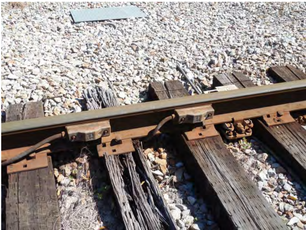
Figure 2-167. Wheel Detectors on Florida Northern Railroad (2015)
