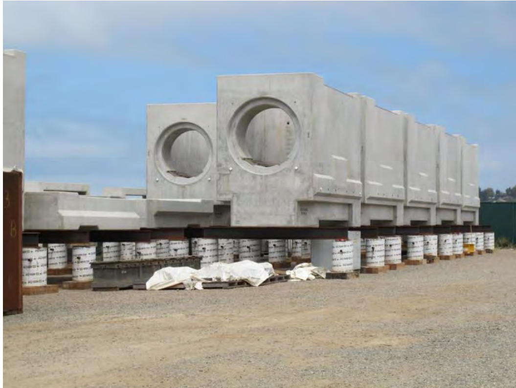
Figure 2-259. Horizontal Storage Modules (2015)
