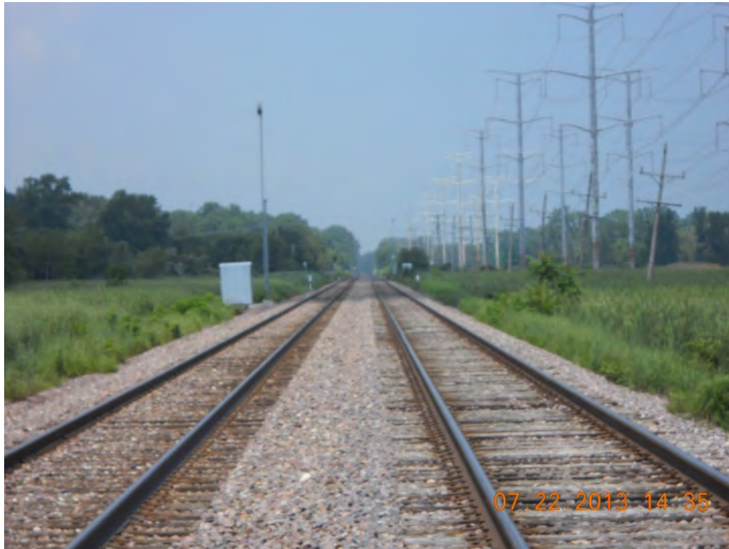
Figure B-16. Union Pacific Mainline at the Zion Site (2013)
