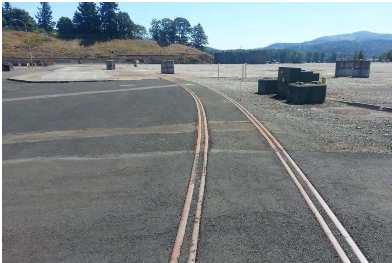
Figure 2-105. Remnants of On-site Rail Spur at Trojan (2013)
