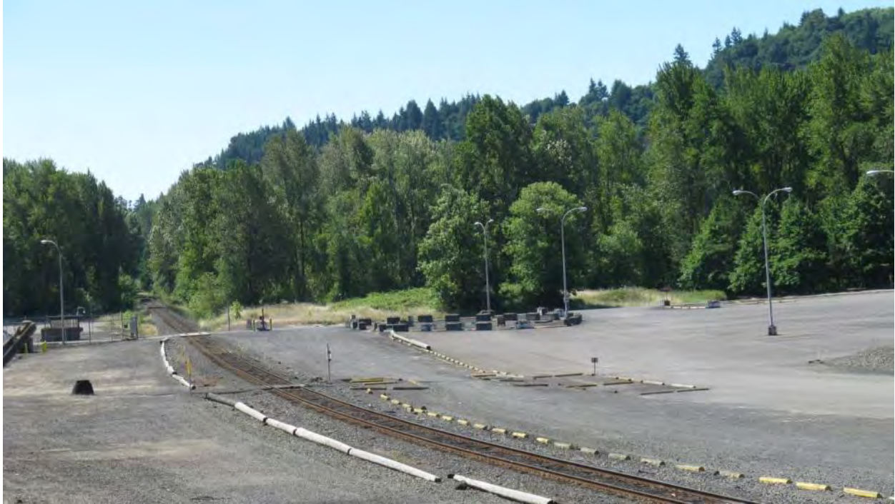
Figure 2-102. Portland and Western Railroad in the Vicinity of the Trojan Site (2013)
