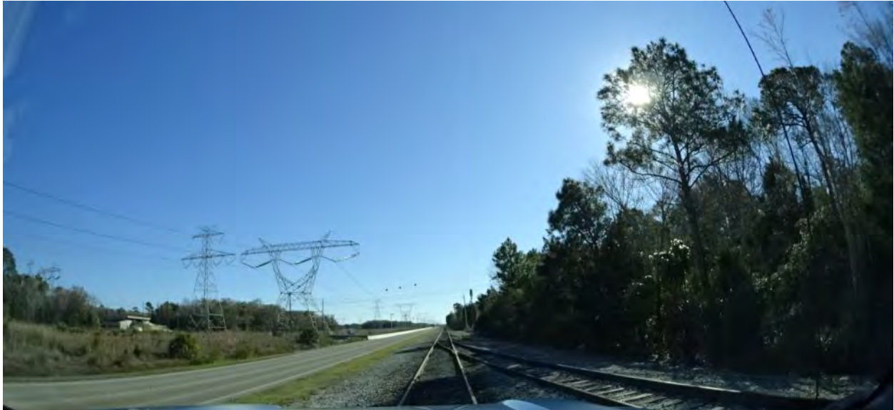
Figure 2-155. Onsite Industrial Rail Spur at the Coal Loop Junction (2015)
