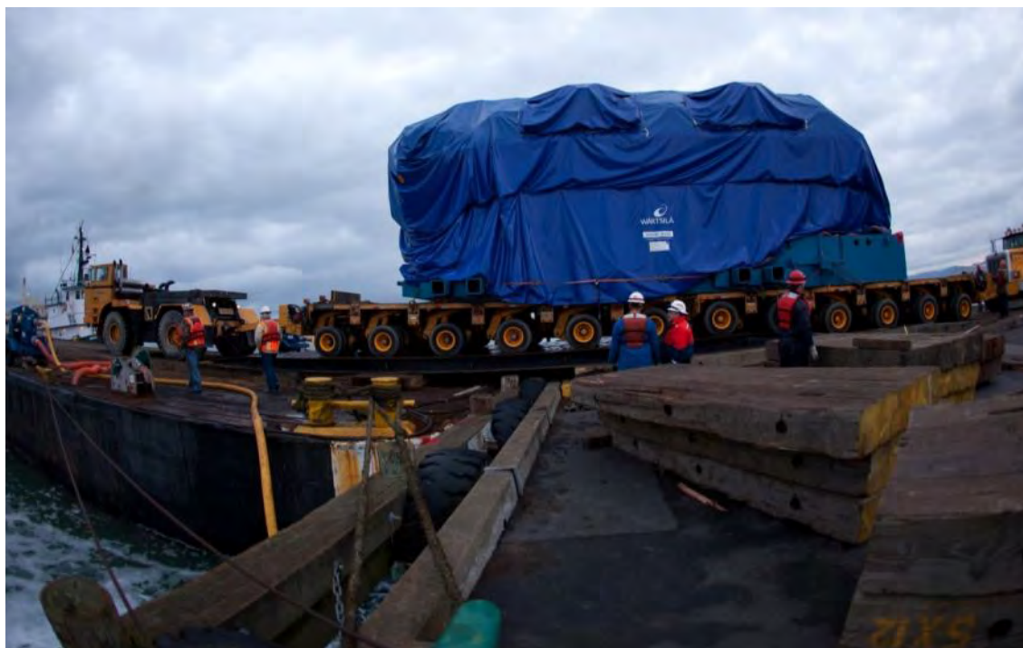
Photo courtesy of Bragg Crane & Rigging Co.
