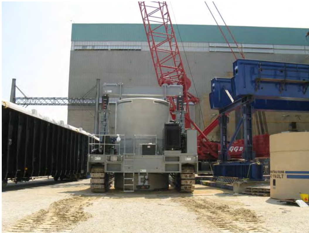
Figure 2-136. Transporter Used to Move Vertical Concrete Storage Casks (2013)
