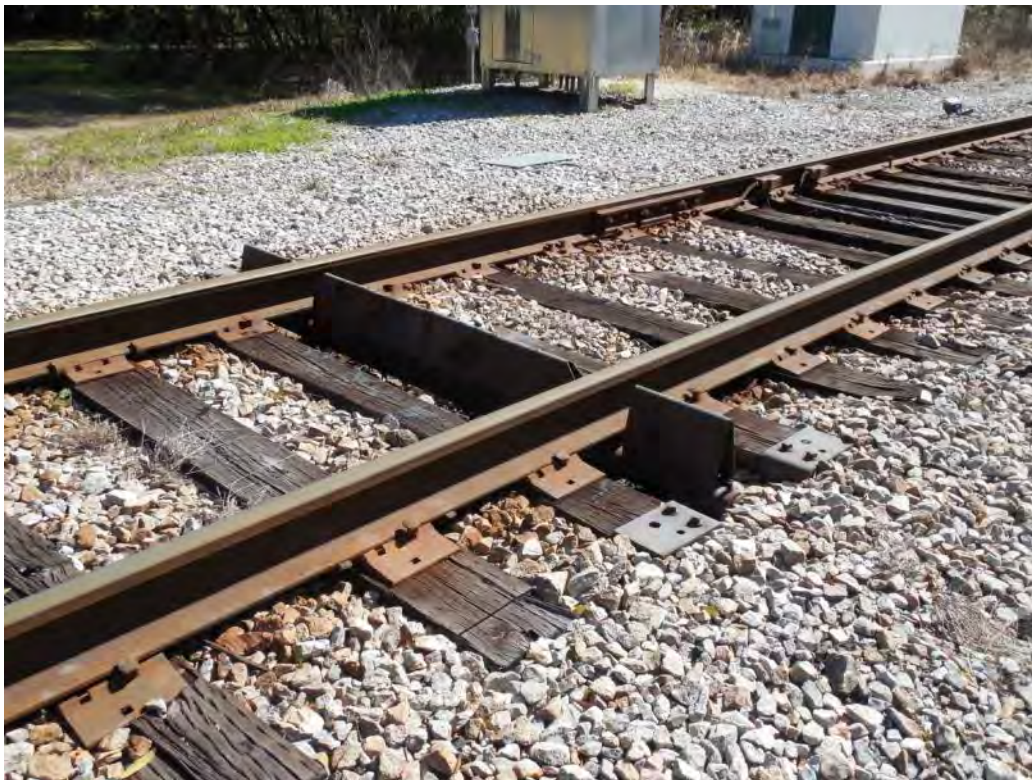
Figure 2-169. Dragging Equipment Detector on Florida Northern Railroad (2015)
