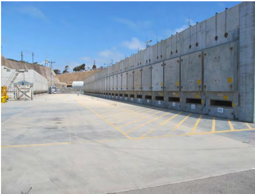
Figure 2-269. Close-up View of San Onofre Independent Spent Fuel Storage Installation (2015)
