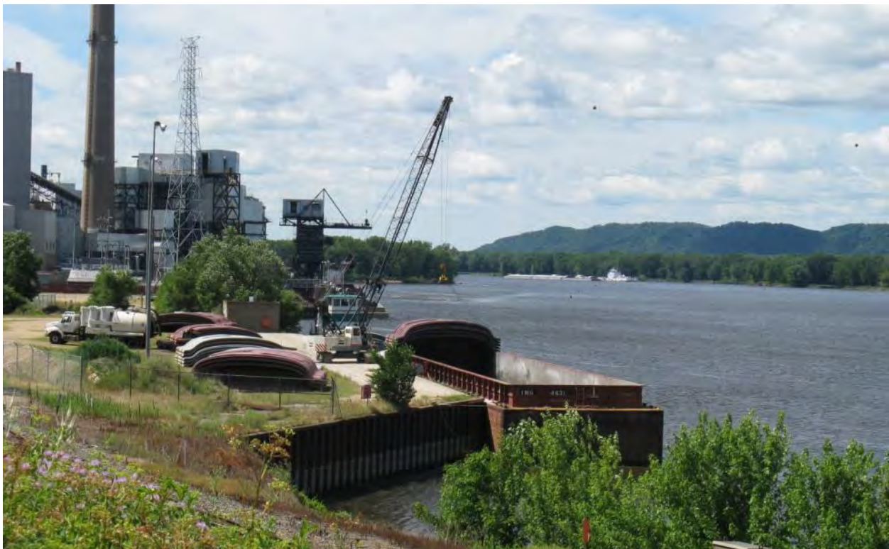
Figure 2-122. Coal Barge at Barge Dock Area at La Crosse Site (2013)
