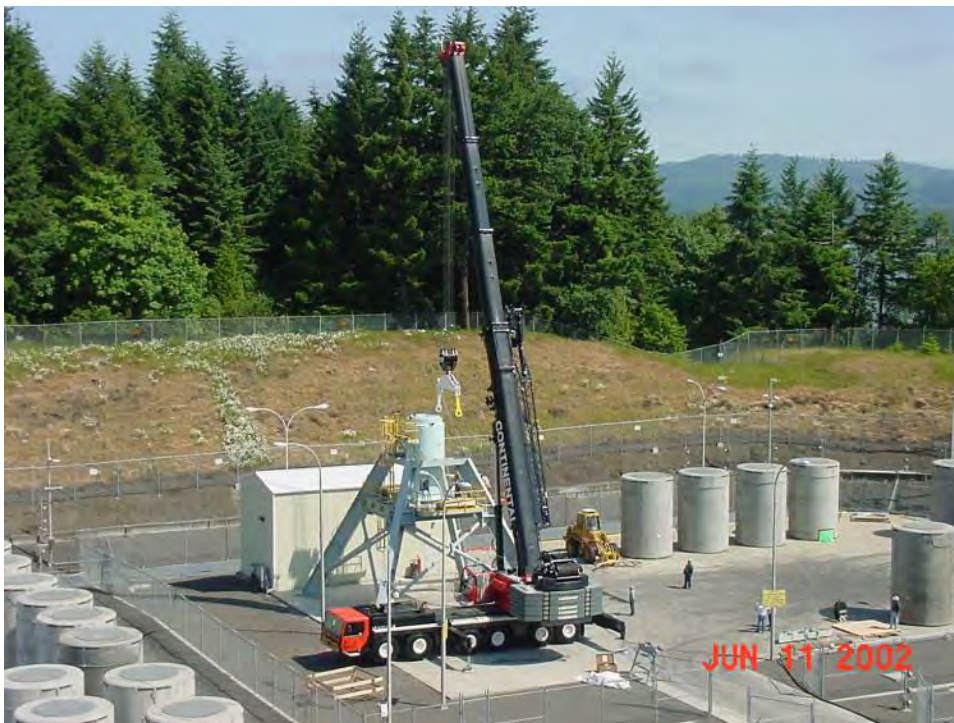
Photo courtesy of Trojan
