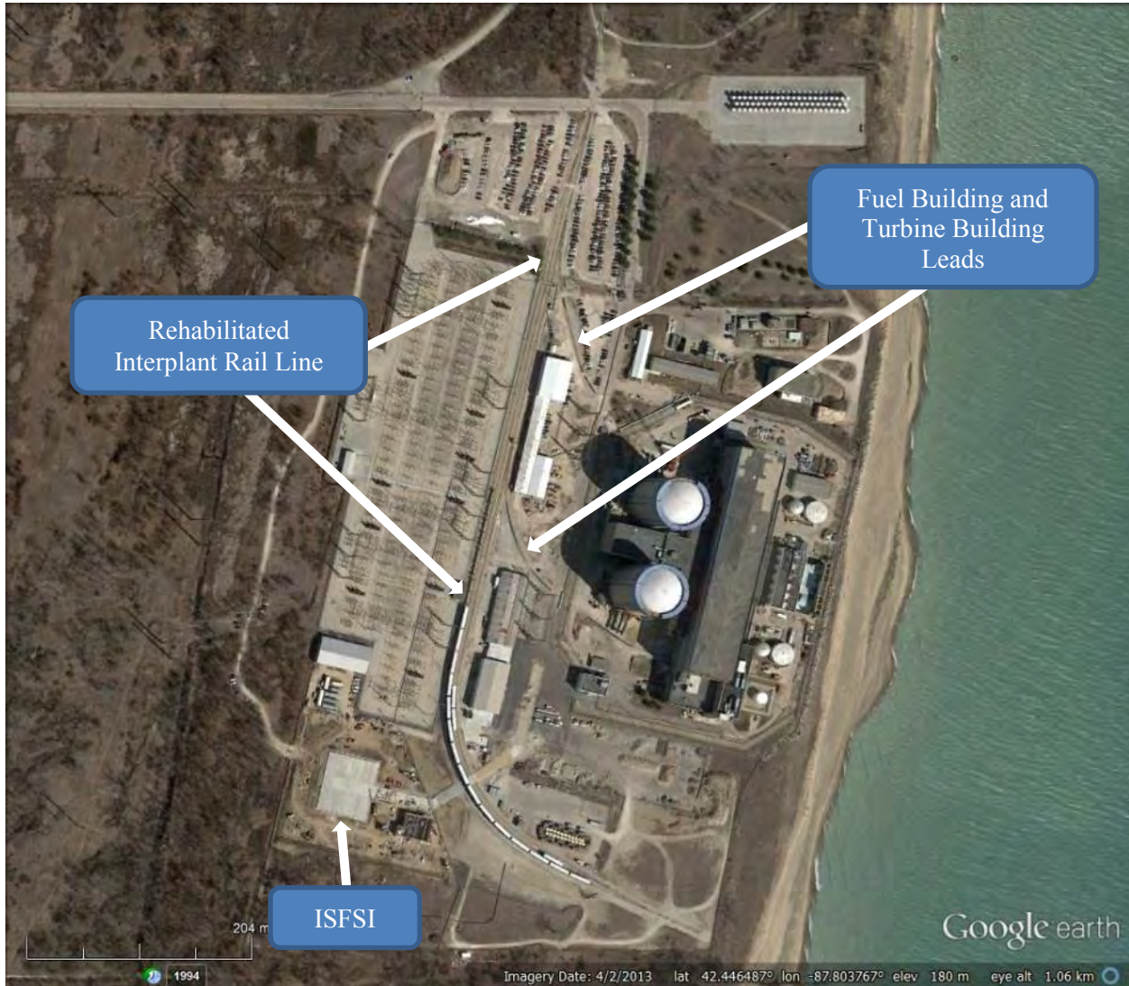
Figure B-21. Satellite view of Zion Site Showing Independent Spent Fuel Storage Installation Pad, the Rehabilitated Interplant Rail Line, and the Leads to the Reactor Containment Building (Google 2015)
