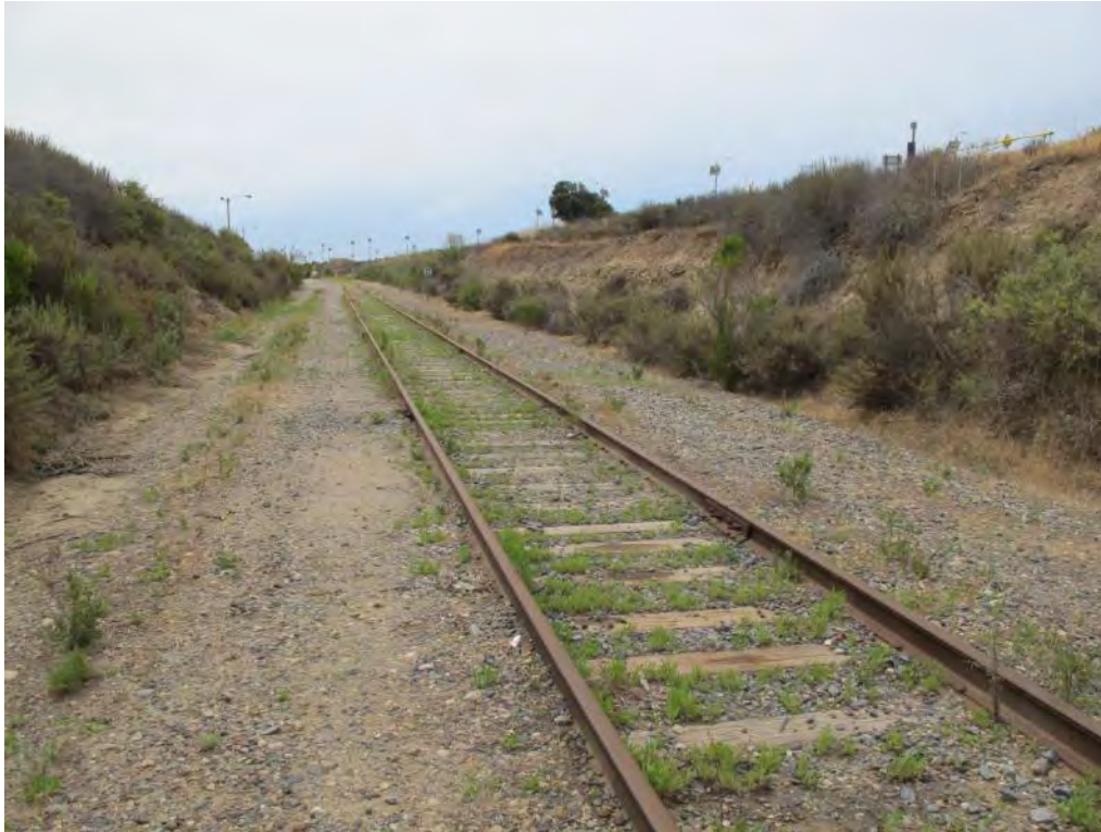
Figure 2-276. Onsite Rail Spur at San Onofre Site (2015)
