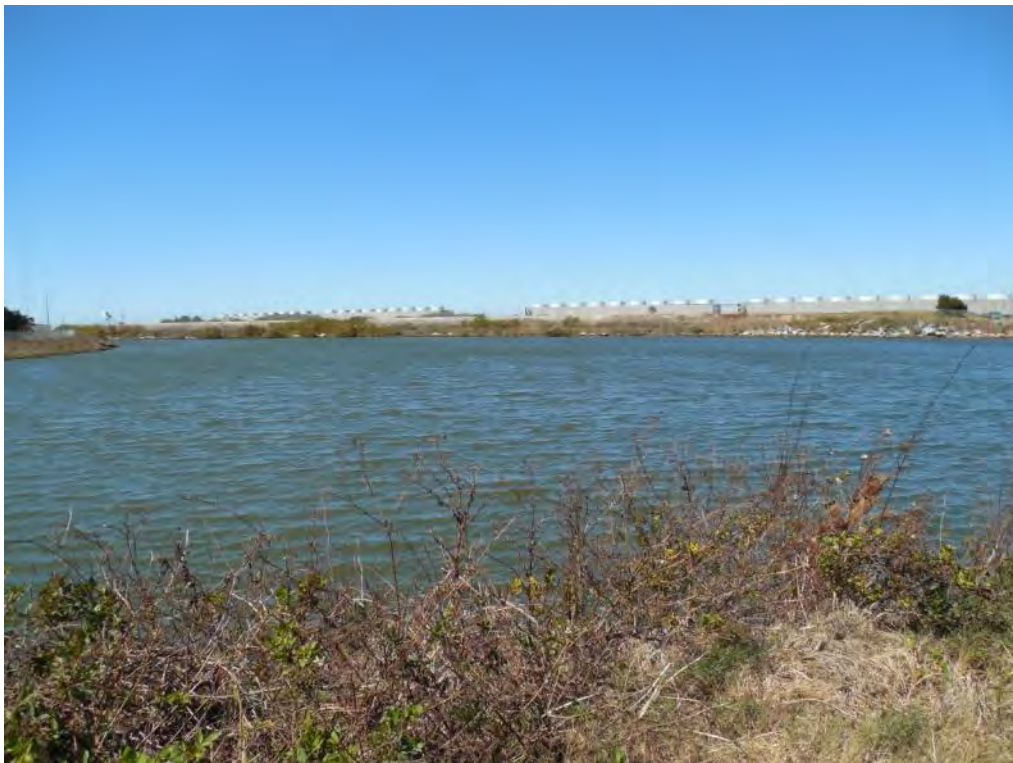
Figure 2-159. Barge Turning Basin (2015)
