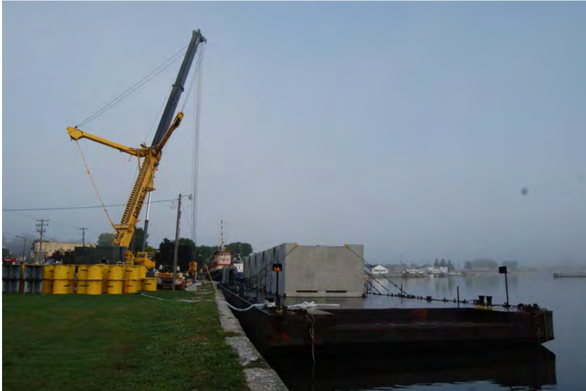
Figure 2-243. Horizontal Storage Modules Being Unloaded from a Barge (2013)
