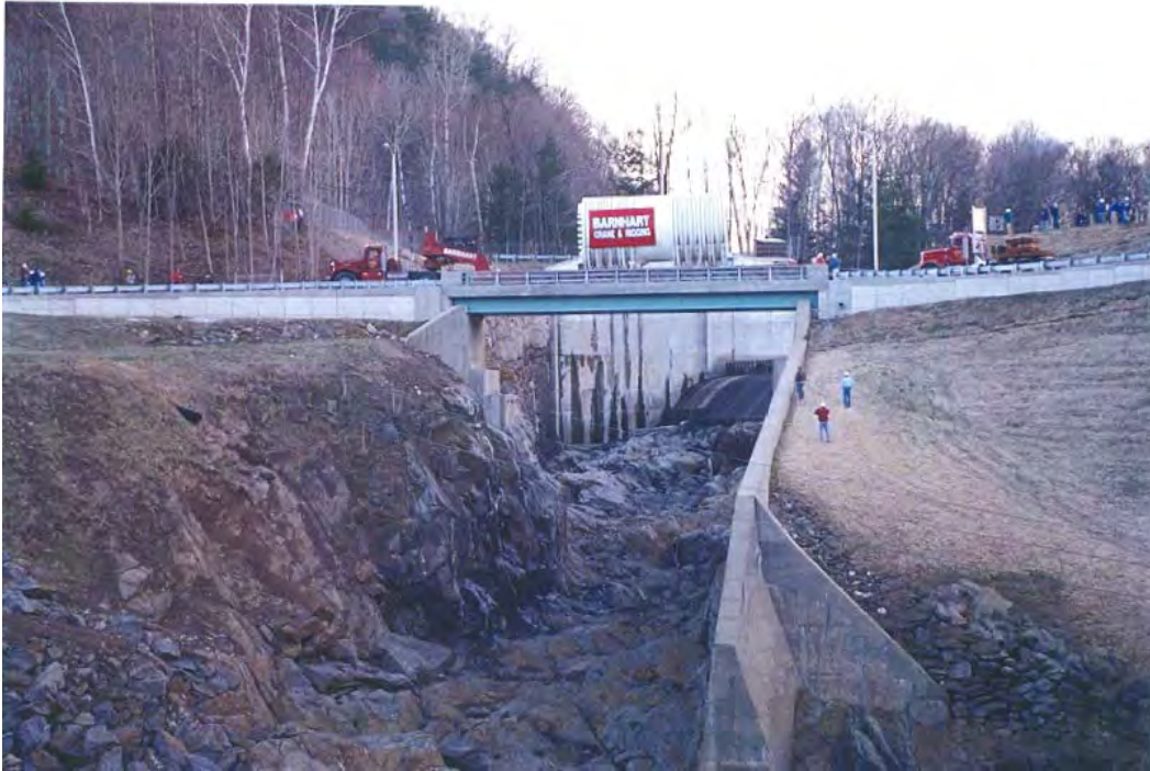
Photo courtesy of AREVA
