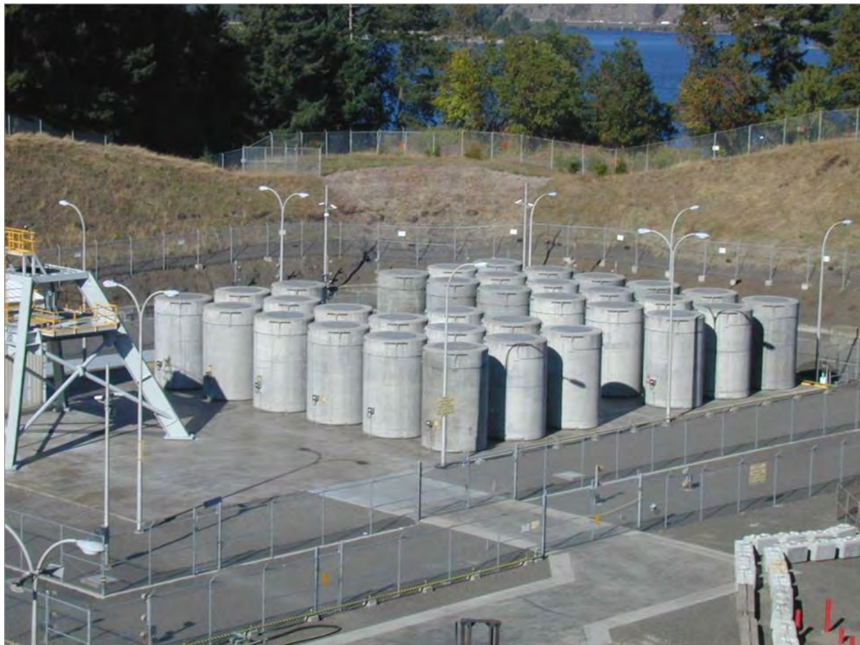
Photo courtesy of Trojan
