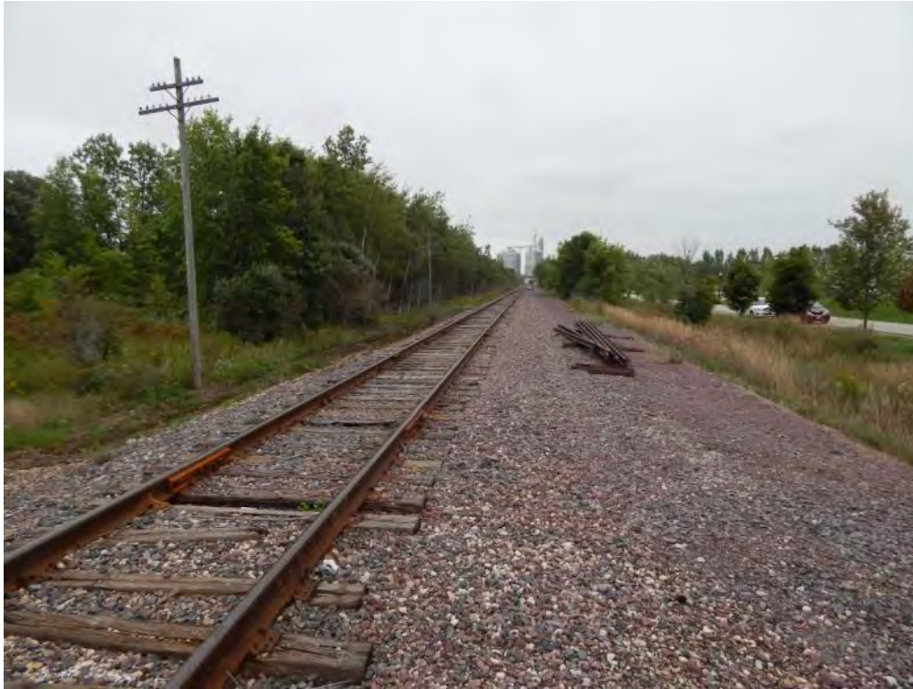
Figure 2-218. Potential Denmark Transload Location (Looking South) (2014)
