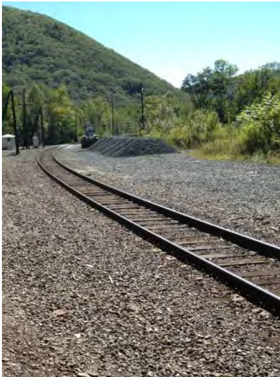
Figure 2-25. Rail Line at East Portal of the Hoosac Tunnel (2012)
