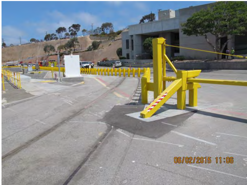
Figure 2-275. Onsite Rail System and Vehicle Barrier near Independent Spent Fuel Storage Installation at San Onofre Site (Looking Northeast) (2015)
