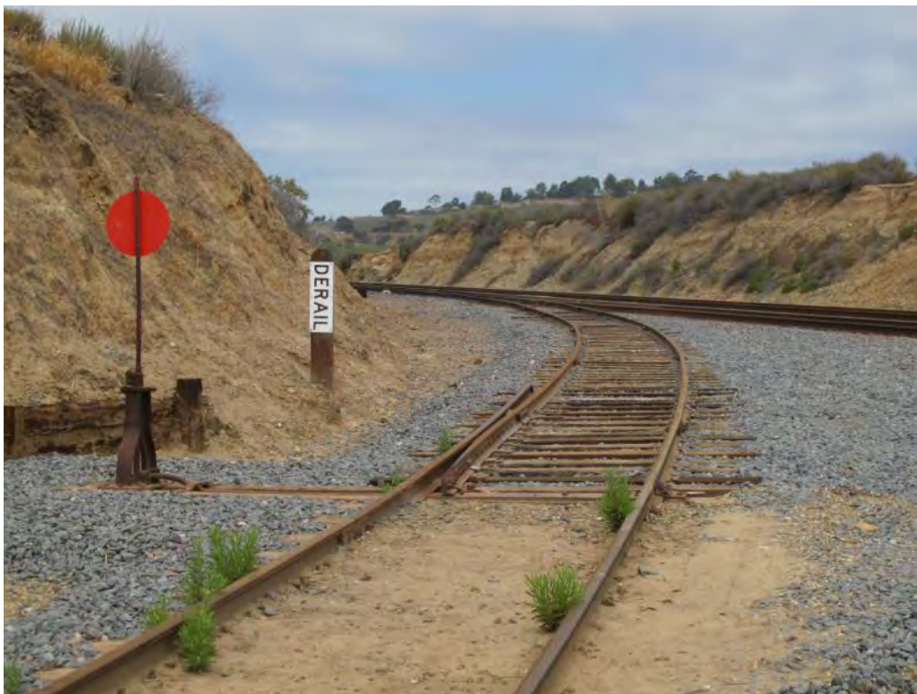
Figure 2-277. Junction of Onsite Rail Spur with Mainline at San Onofre Site (2015)
