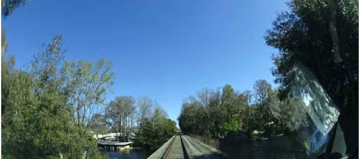
Figure 2-166. Florida Northern Railroad Bridge (2015)
