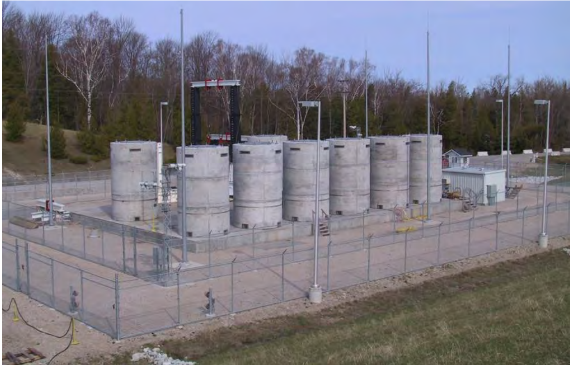
Photo courtesy of Big Rock Point
