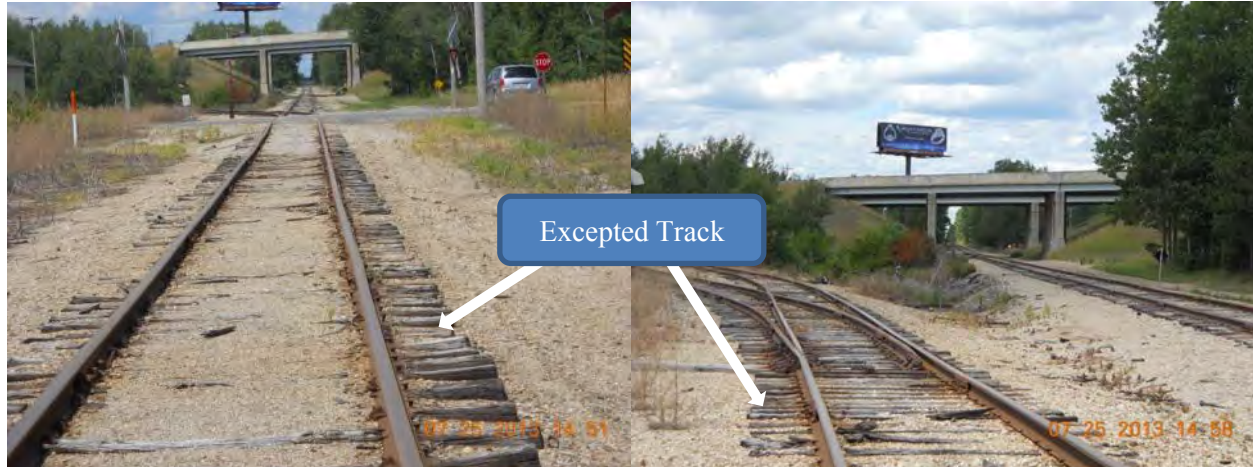
Figure B-8. Track Condition in the Vicinity of Gaylord Transload Location (Looking North) (2013)
