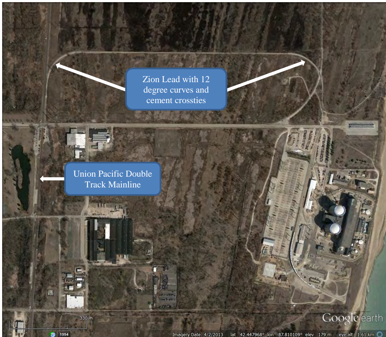
Figure B-22. Satellite View of the Zion Lead and the Union Pacific Double Track Mainline (Google 2013)
