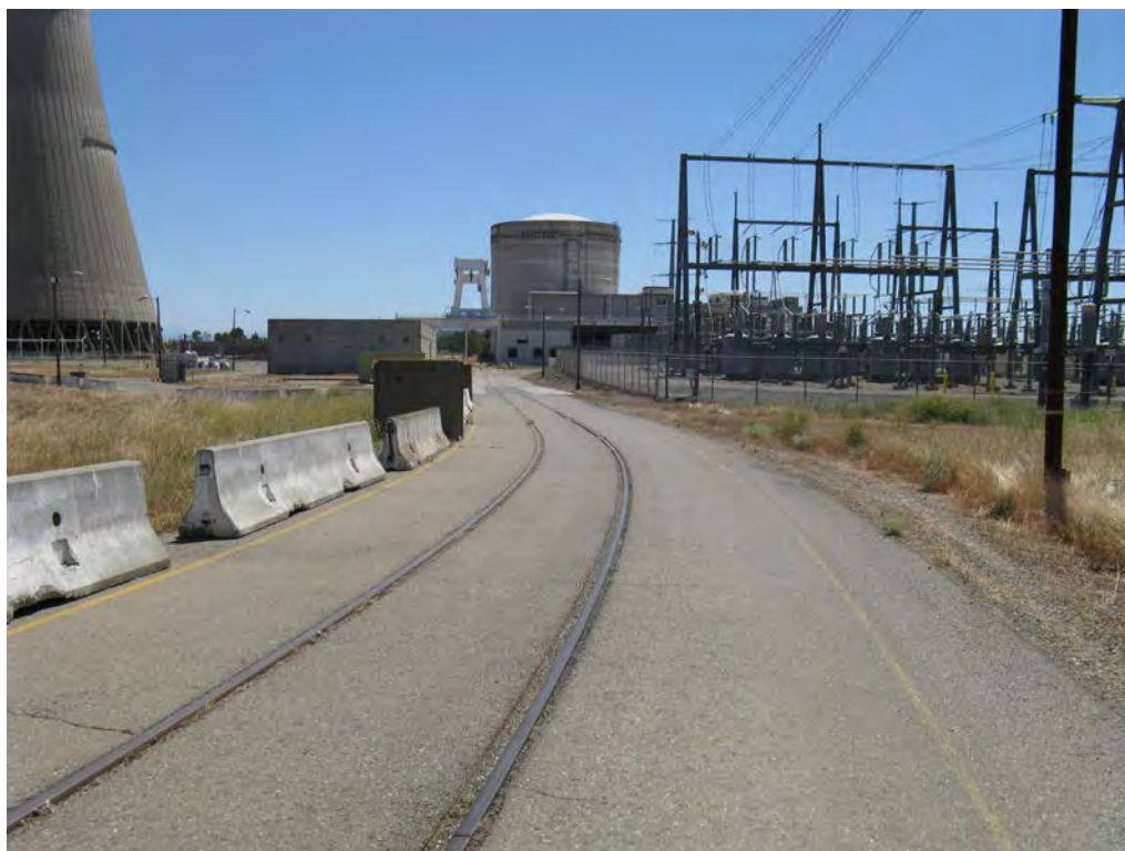
Figure 2-86. On-site Rail Spur Running into Rancho Seco Site
