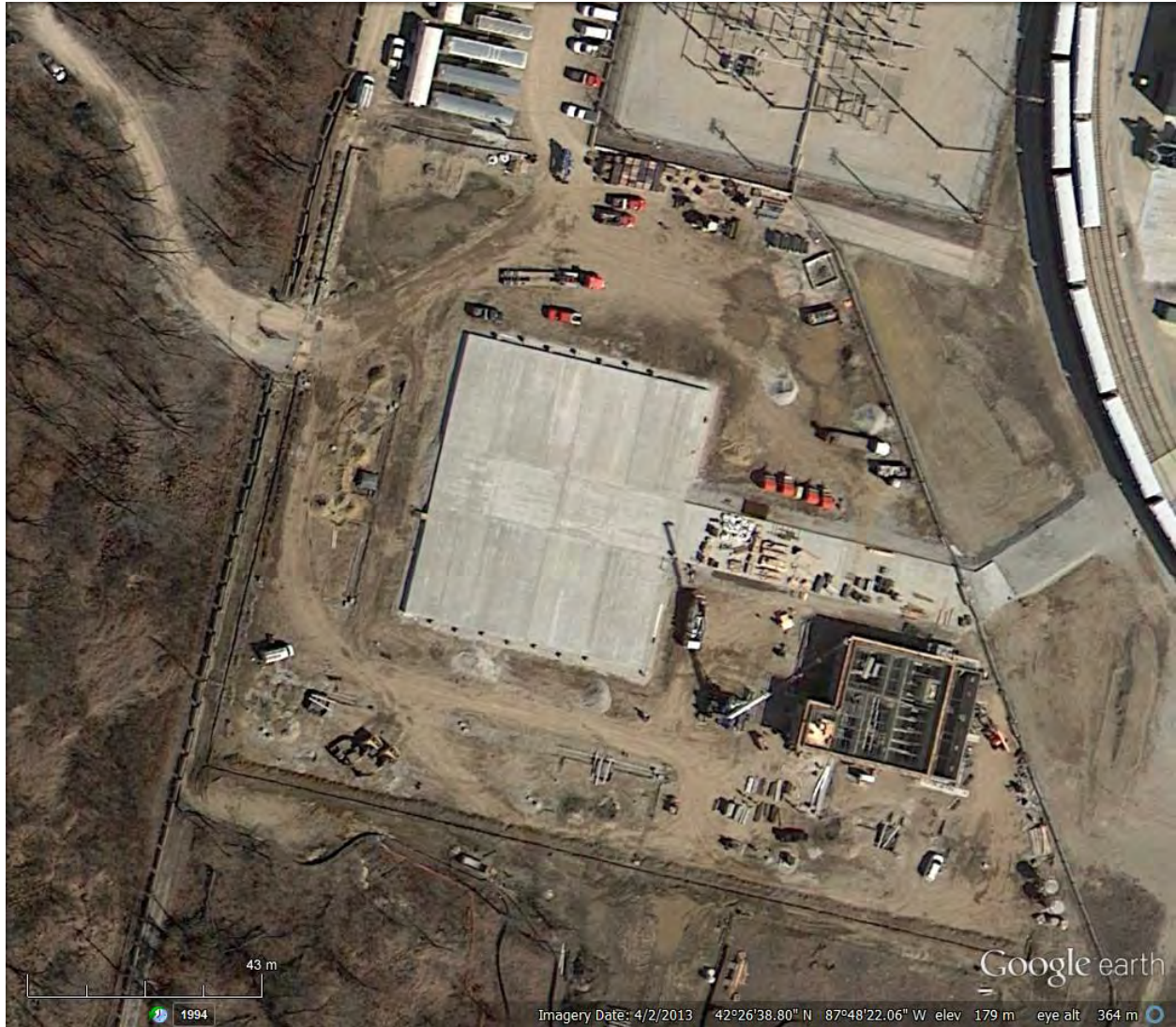
Figure 2-122. Aerial View of Zion ISFSI Under Construction (Google 2013)
