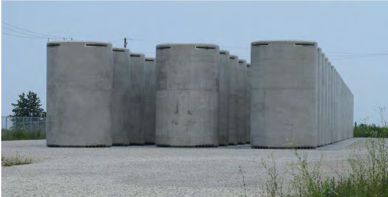
Figure 2-123. Vertical Concrete Storage Casks Staged at Zion
