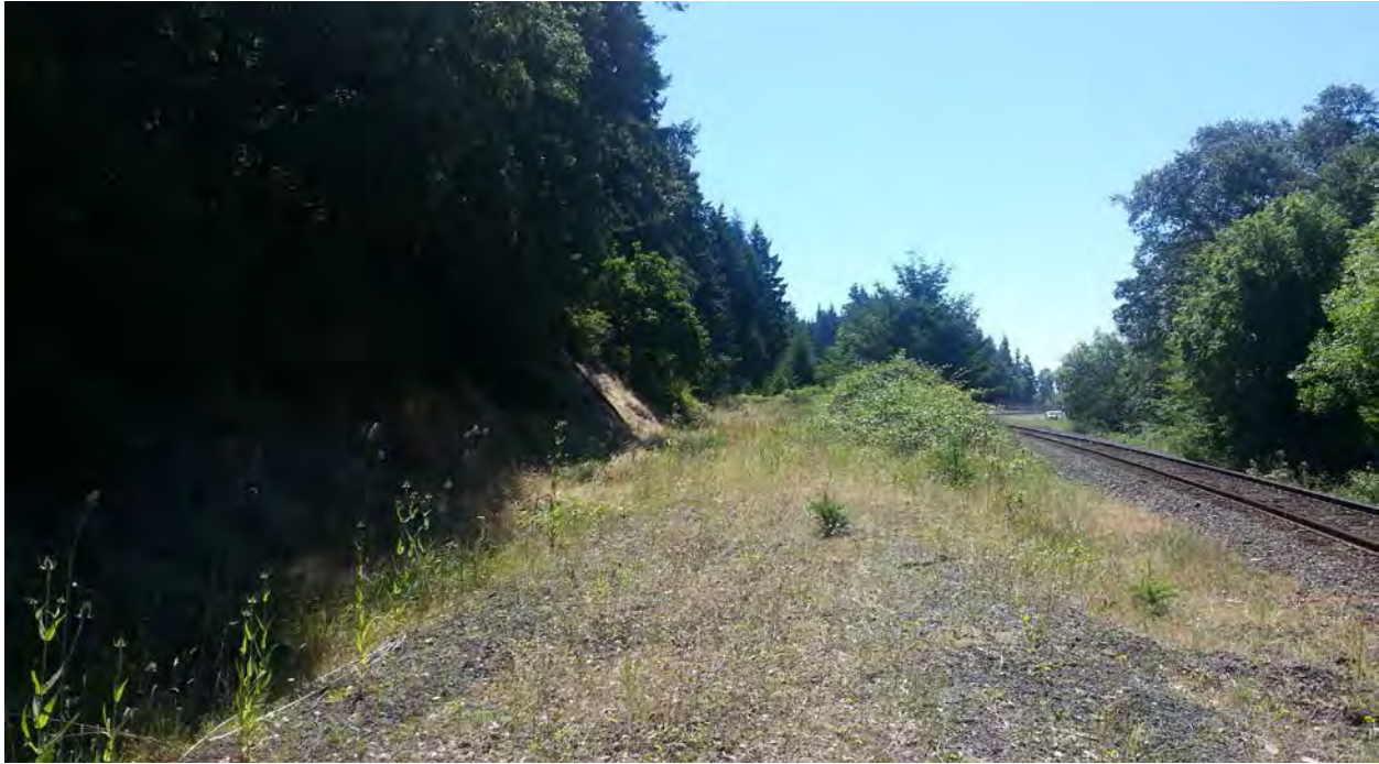
Figure 2-98. Former Trojan Rail Spur Railbed
