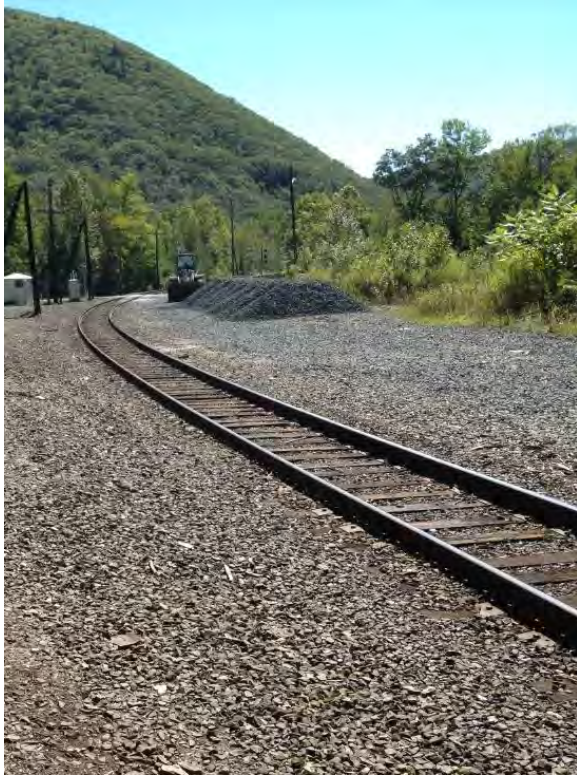
Figure 2-24. Rail Line at East Portal of the Hoosac Tunnel
