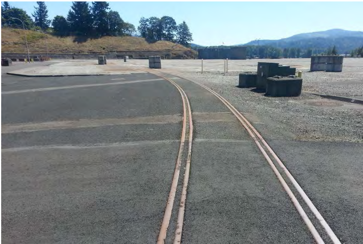
Figure 2-99. Remnants of On-site Rail Spur at Trojan
