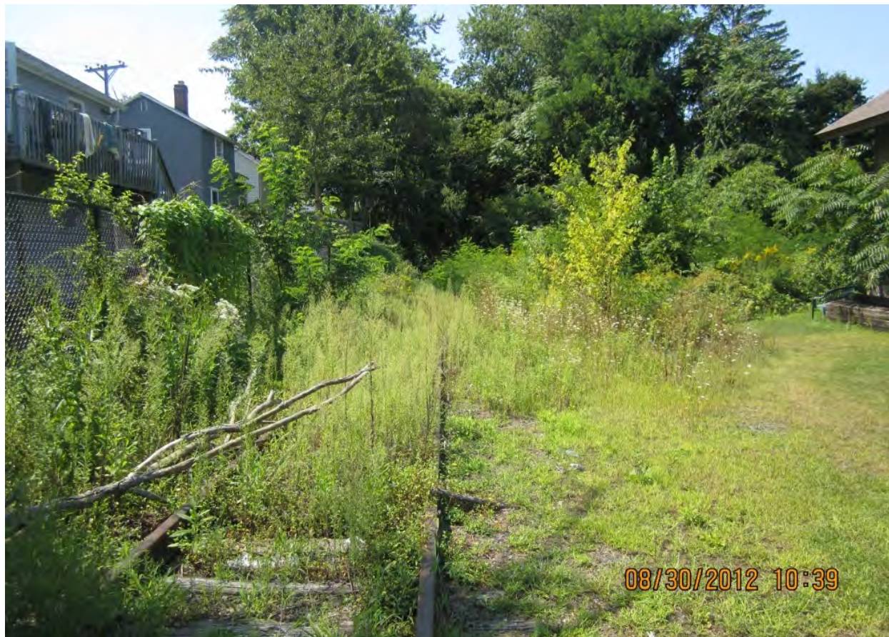
Figure 2-36. Conditions at the End of the Portland Rail Spur in 2012
