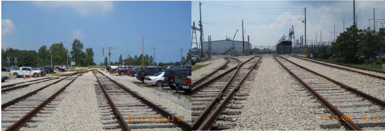
Figure B-19. Zion Site Plant Lead
