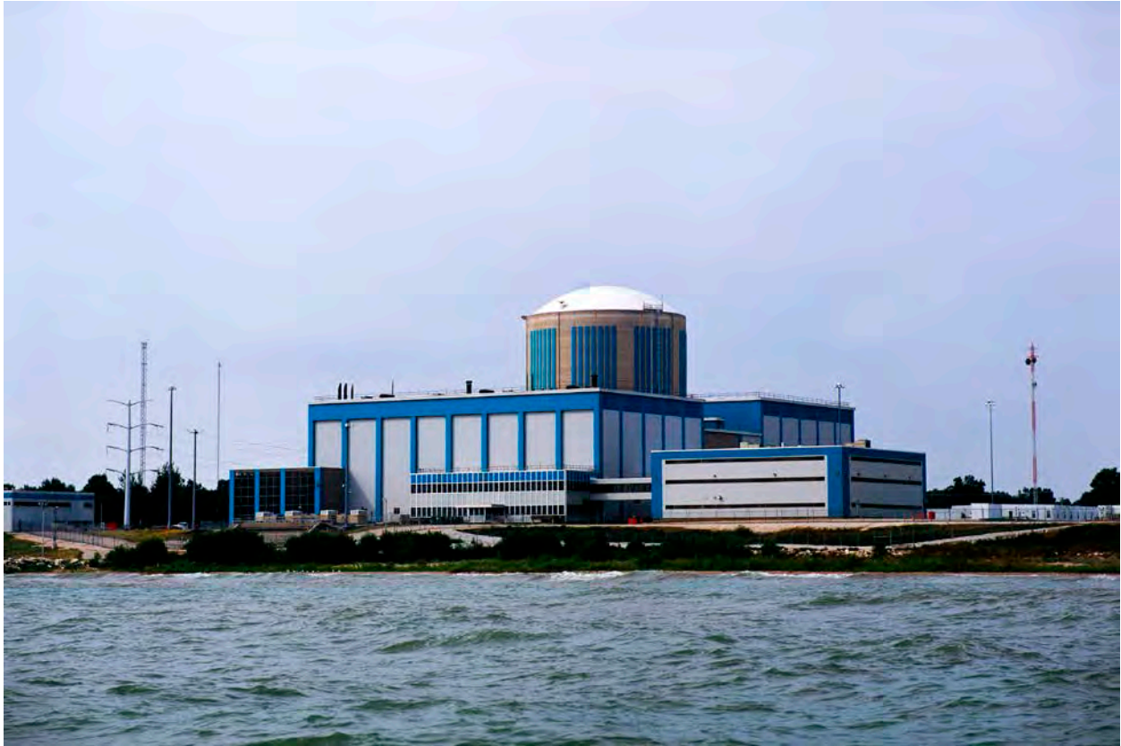
Photo courtesy of Dominion Energy
