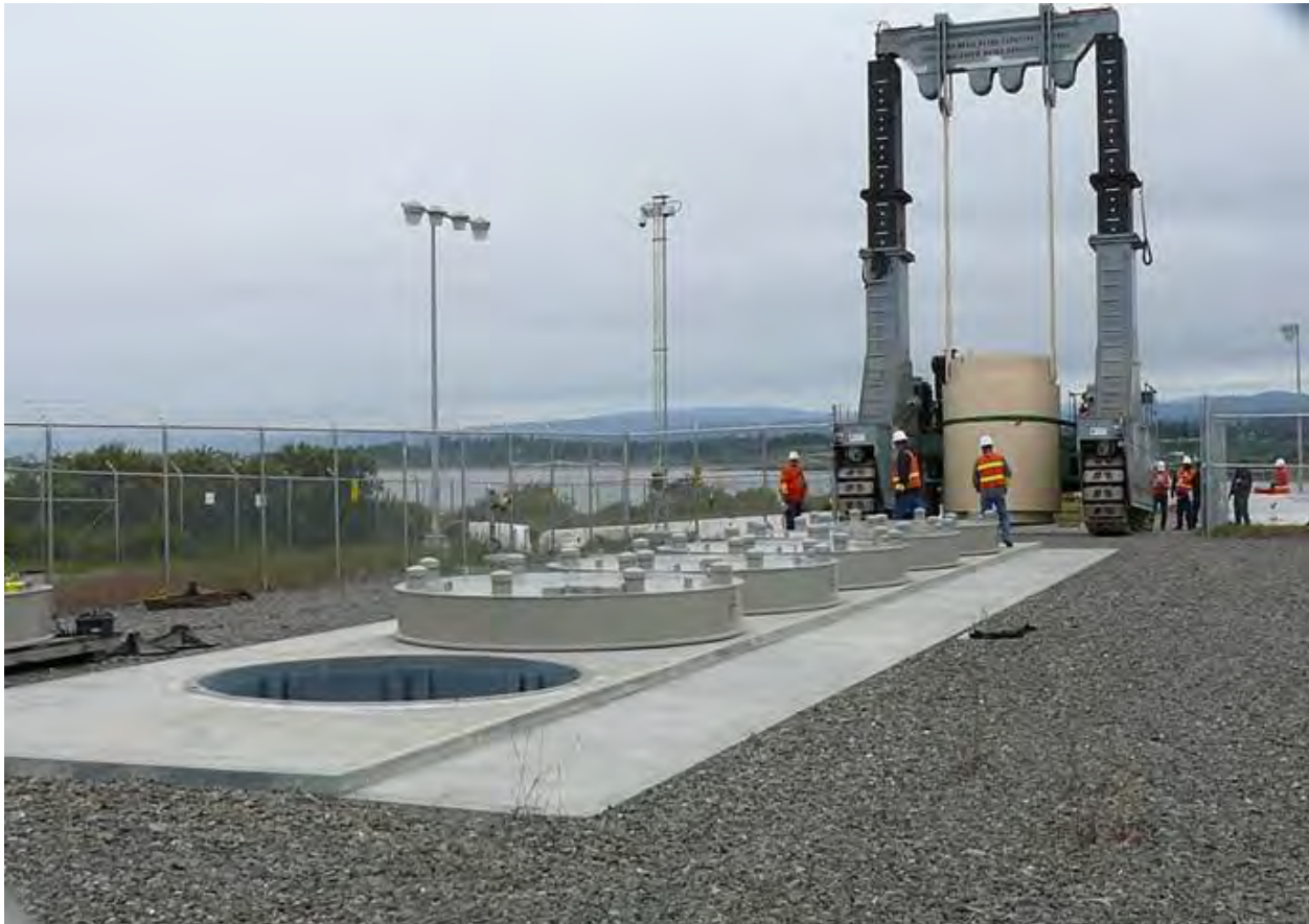
Photo courtesy of Humboldt Bay
