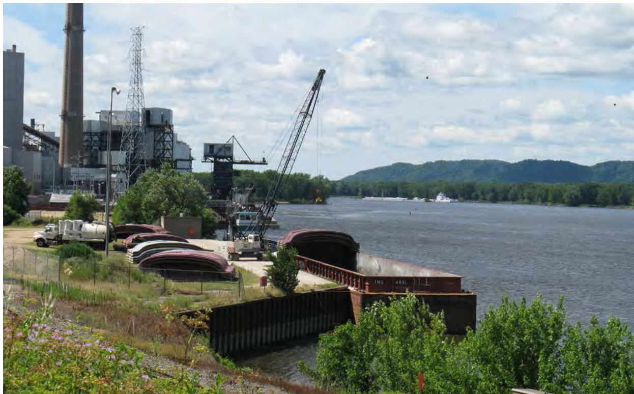
Figure 2-115. Coal Barge at Barge Dock Area at La Crosse Site
