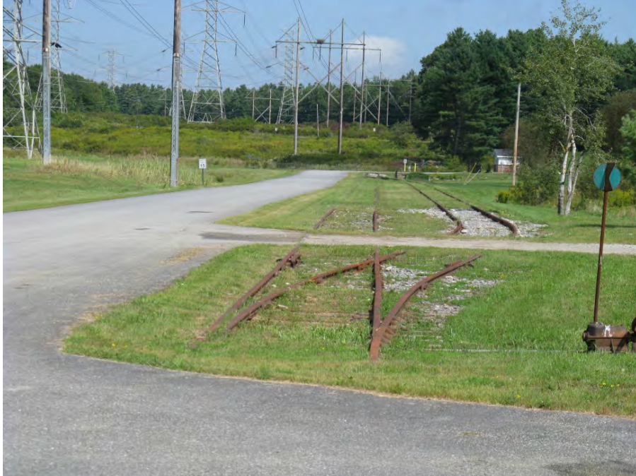
Figure 2-12. Paved-over Railroad Tracks at the Maine Yankee Site
