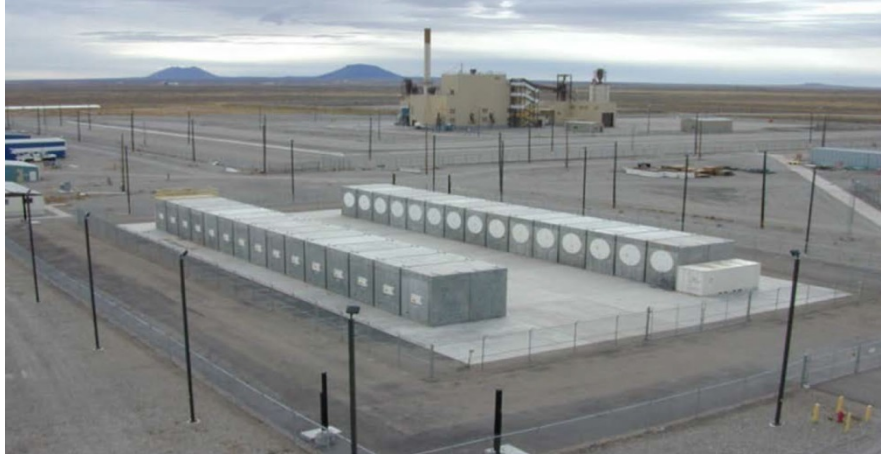
Figure 3.6. Photograph of a NUHOMS Storage Facility at INL (photograph courtesy of INL)
