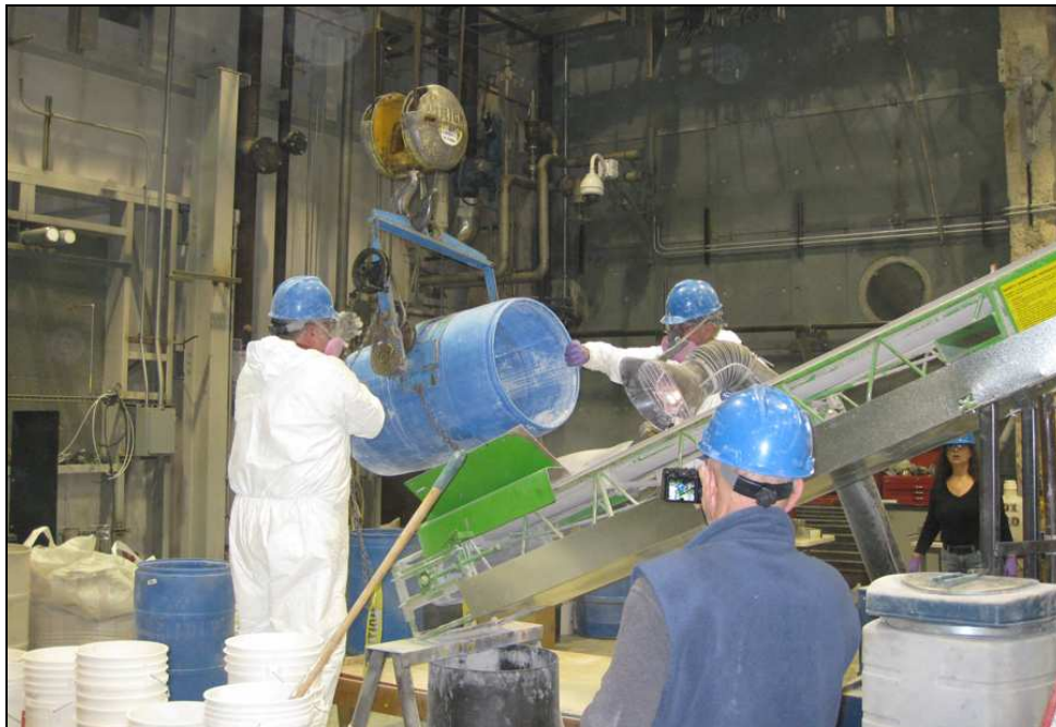
Figure 7-19. Dry material fed using the overhead crane.
