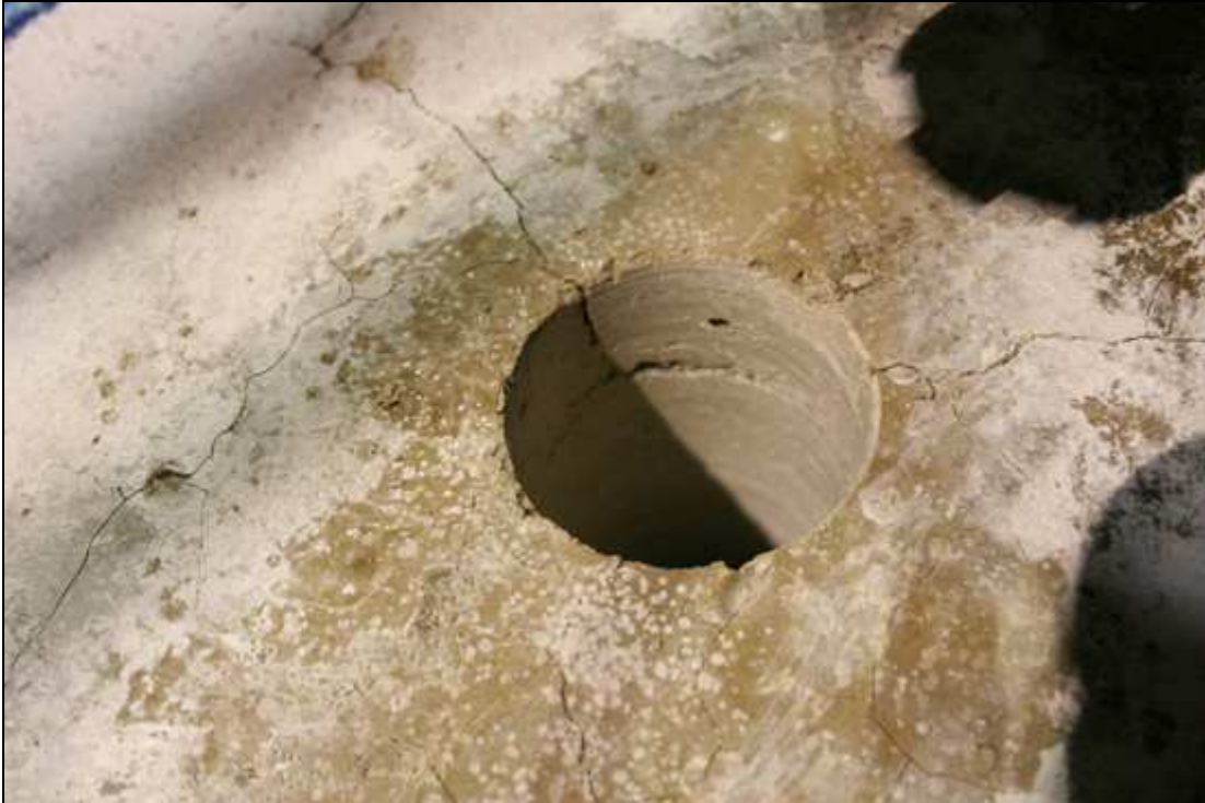
Figure 9-13. Interior of the right hand side of Ceramicrete Sample #6 after coring.
