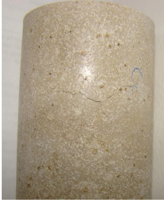
Figure 5.10. Preexisting Crack Observed in Ceramicrete Specimen
