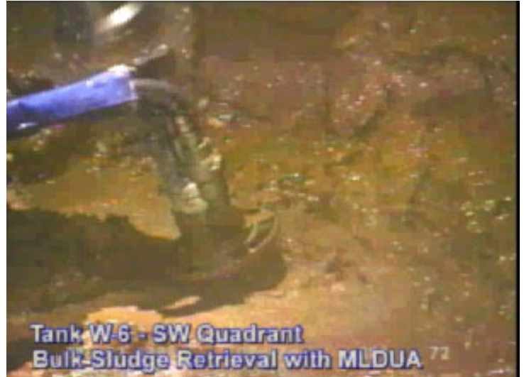
Figure 4.3 High-pressure scarifier and air conveyance (left) and confined sluicing end-effector and jet pump conveyance (right)
