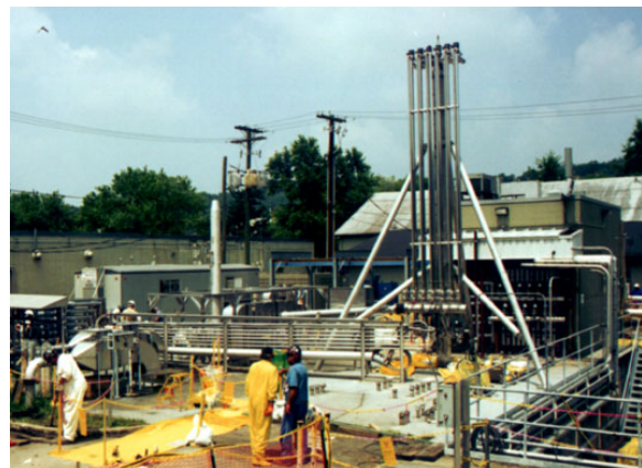
Figure 5.2 View of Pulse-Air mixer before deployment in tank W-9 and pulsed jet fluidic mixer at Bethel Valley Evaporator Service Tanks
