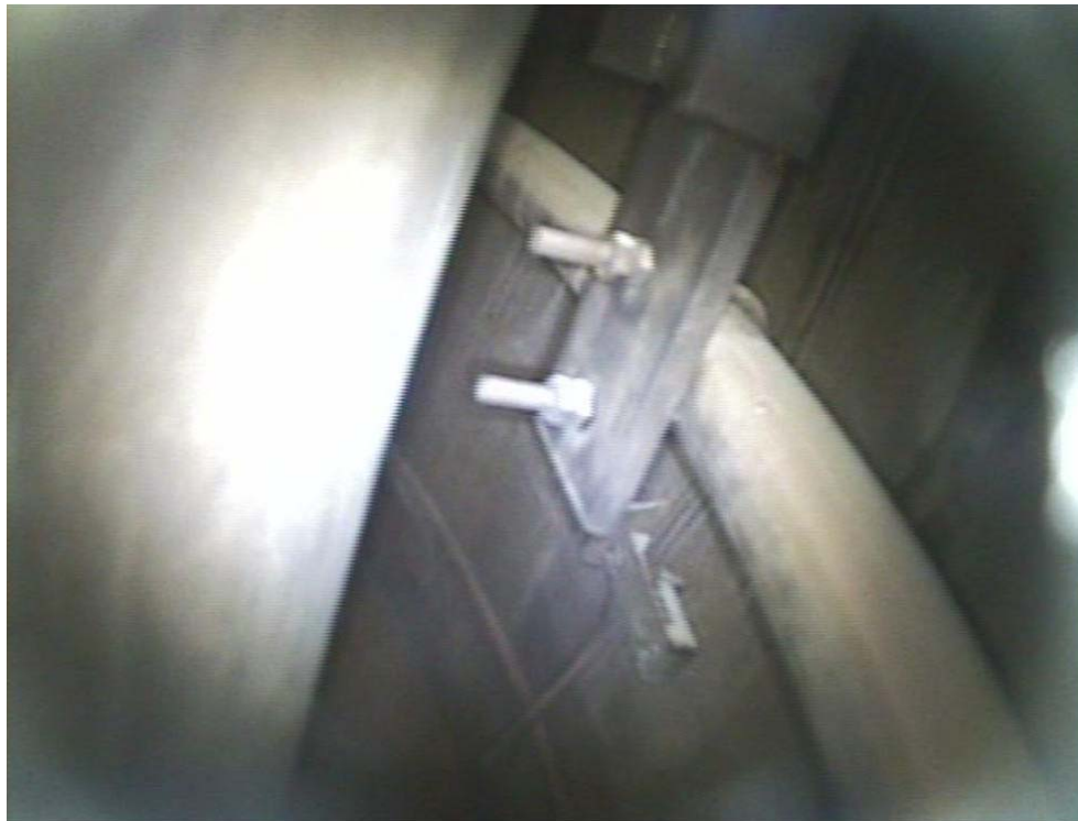
Figure 13.6. The Steam Ring and Bracket in Tank T01A After IW Cleaning
