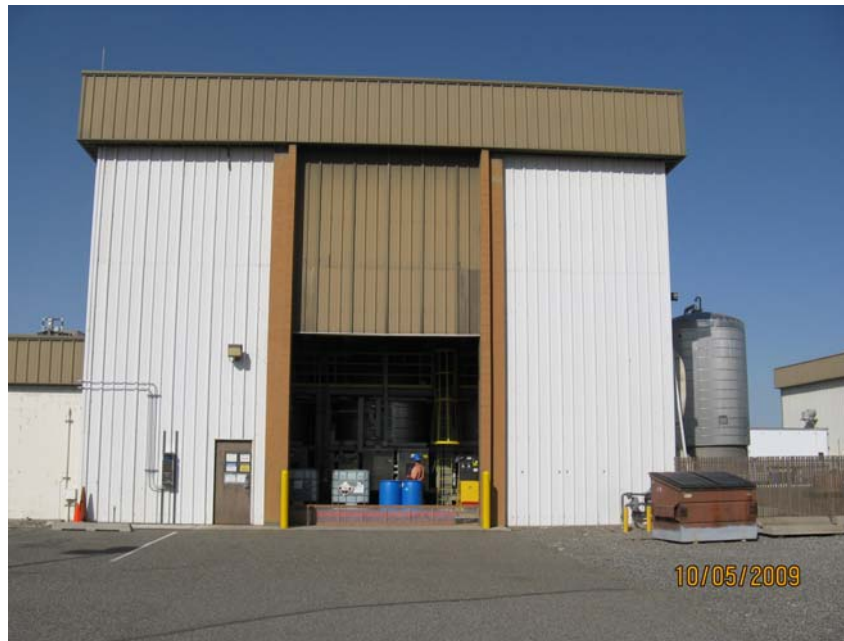
Figure 4.2. A Majority of the PEP Skids Were Moved into PDL-W and Assembled into the Two-Story Structure (looking North)
