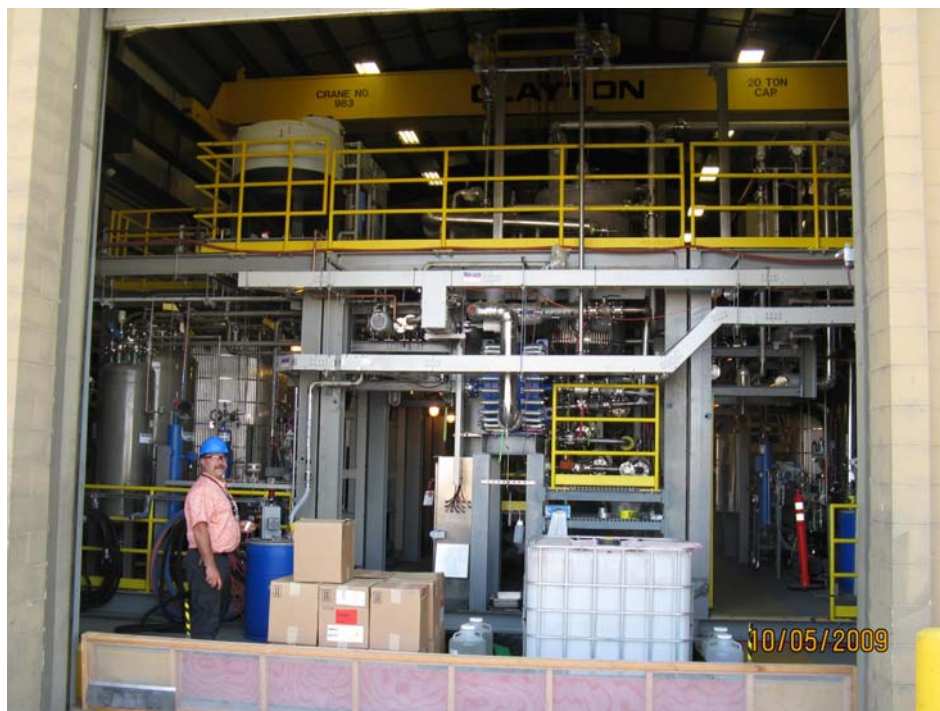
Figure 4.4. The PEP as Viewed Through the North Rollup Door on PDL-W
