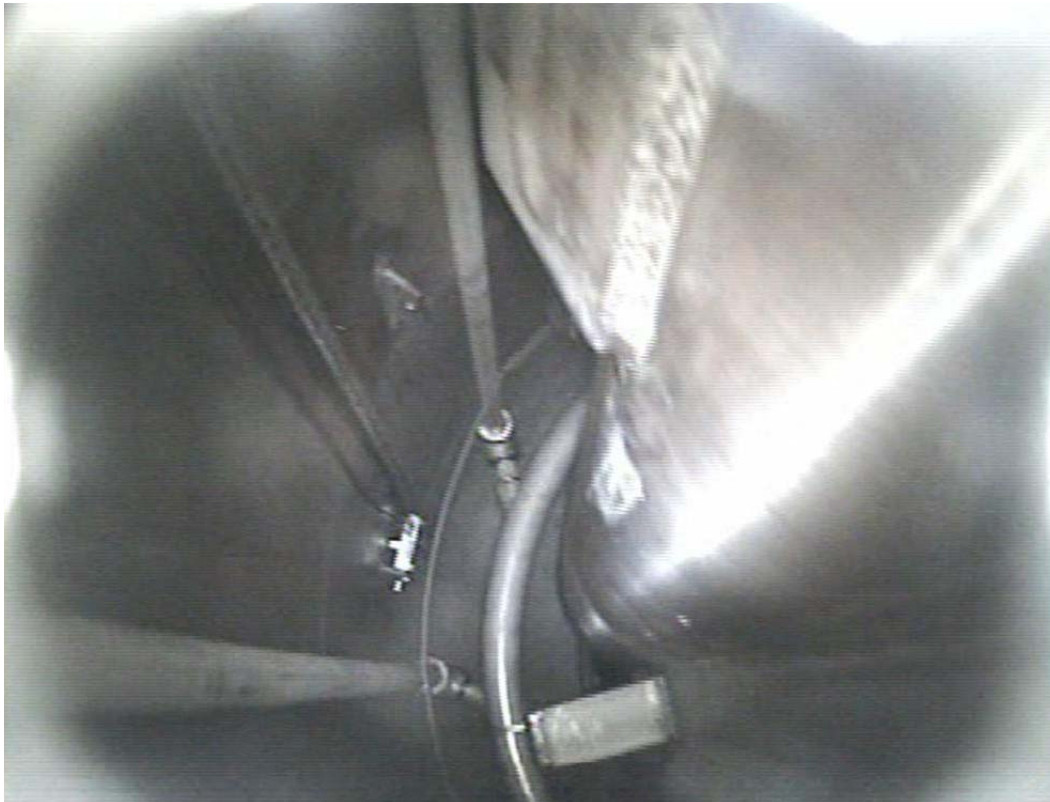
Figure 13.7. Tank T02A After the Prototypic Nitric Acid Cleaning. This is the portion of the tank that was exposed to acid during the cleaning process.
