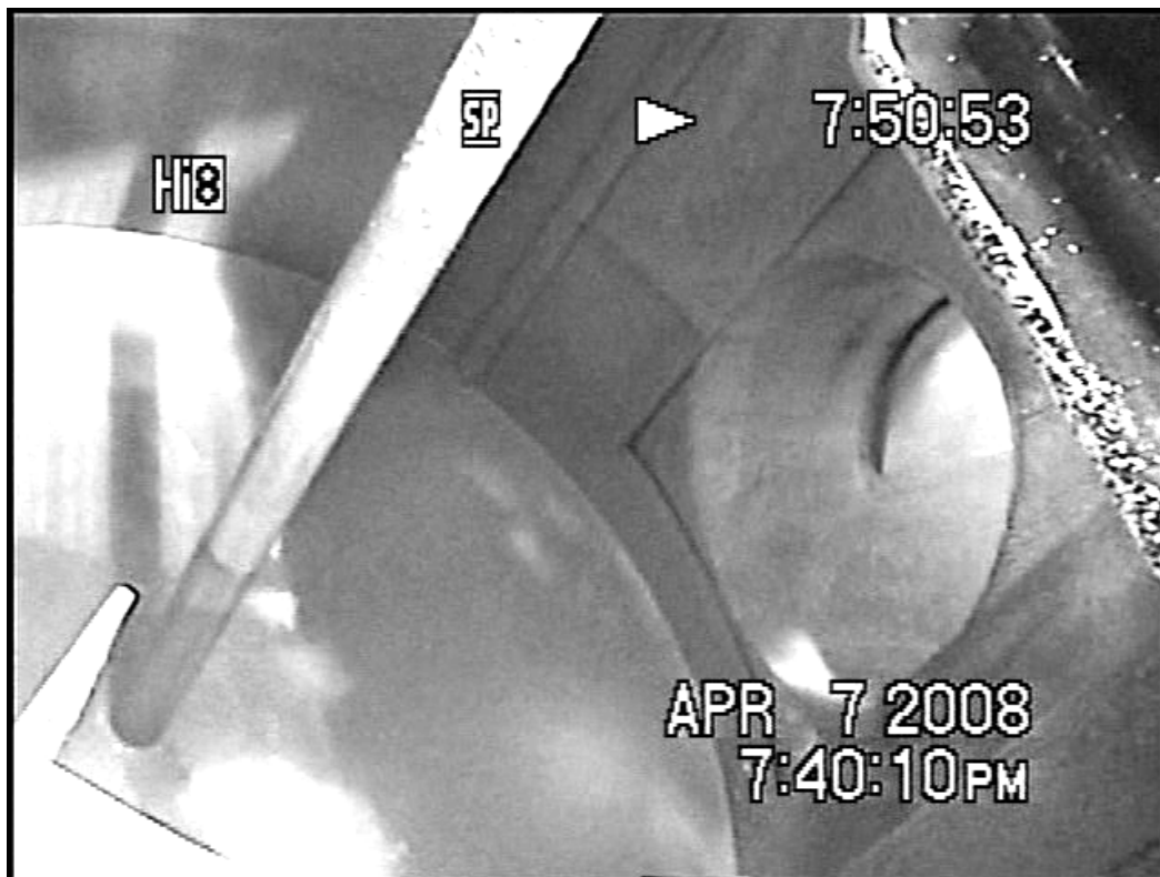
Figure 8.10. Pipe Entrance from Upstream Reservoir
