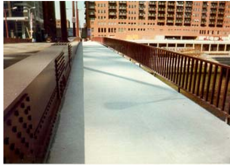
Ceramicrete Bridge Deck, Chicago, Illinois
