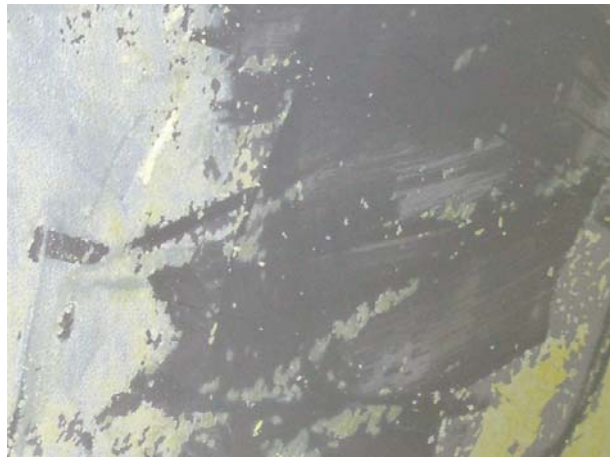
Figure 4.17. Close-Up of Partially Scraped and Vacuumed Aspigel-Treated Panel
