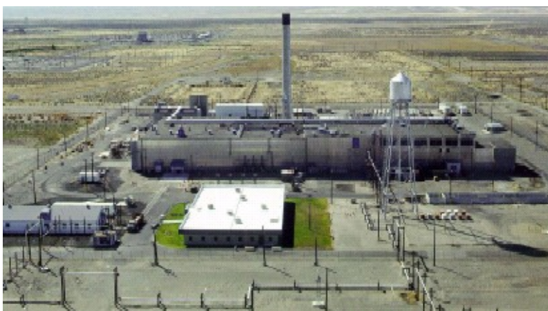
Figure 1.1. Hanford's Plutonium Finishing Plant (Richland 2005)
