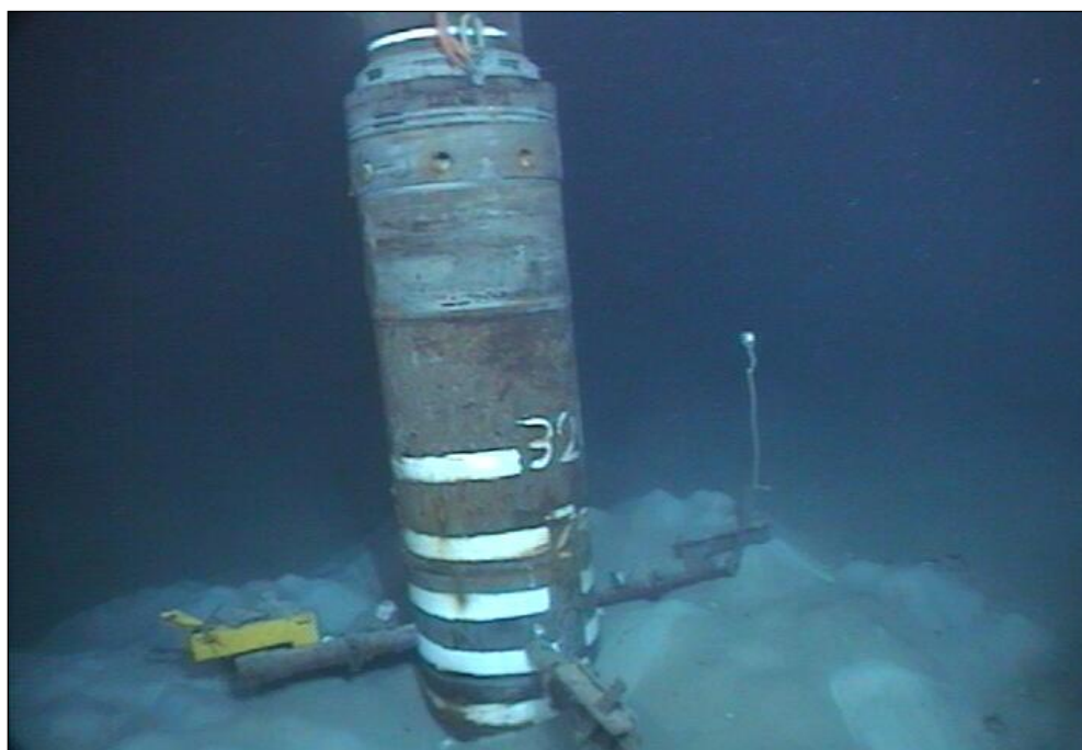
Figure 10-89. Chevron wellhead observed during JII-282, at AC818.
