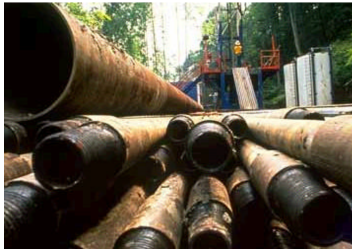
Figure 7.1. Natural Gas Pipes.
