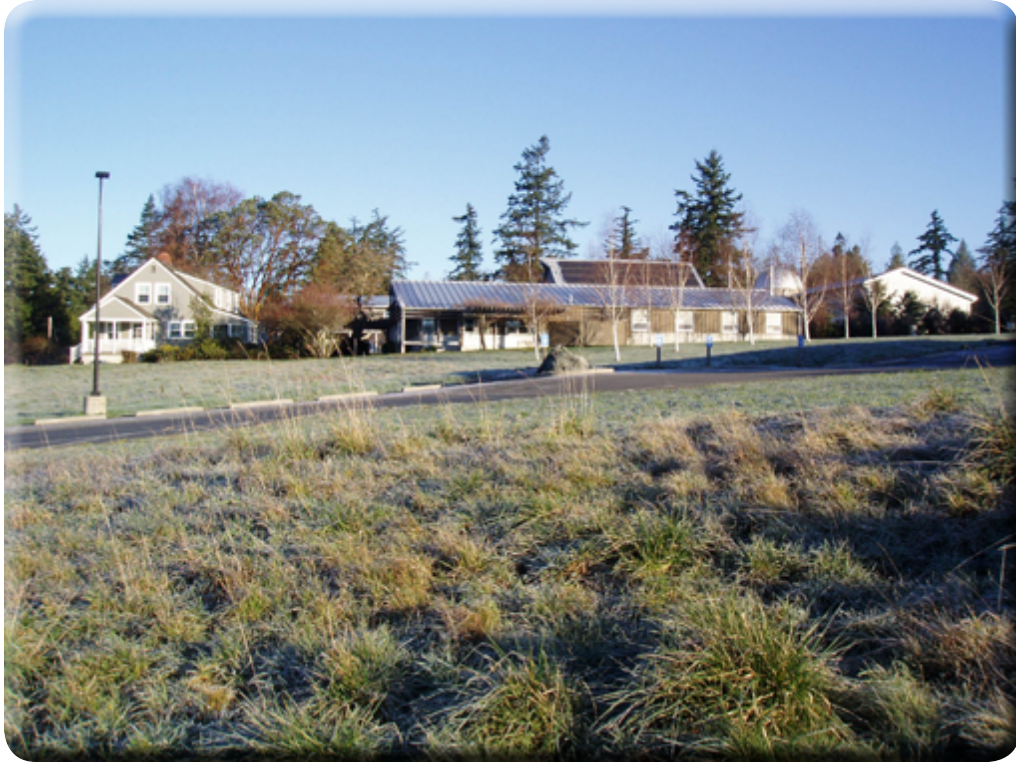
Figure 10.6 Breazeale House (left), Research Laboratory (middle) and boat garage (right).
