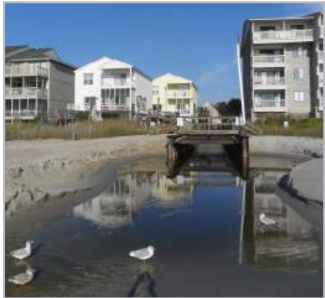
Swashes are relic tidal creeks in the Grand Strand, which now serve as conduits for stormwater into the ocean. Scientists are working with local decision-makers to better understand the role of swashes in hypoxia formation in coastal waters.
