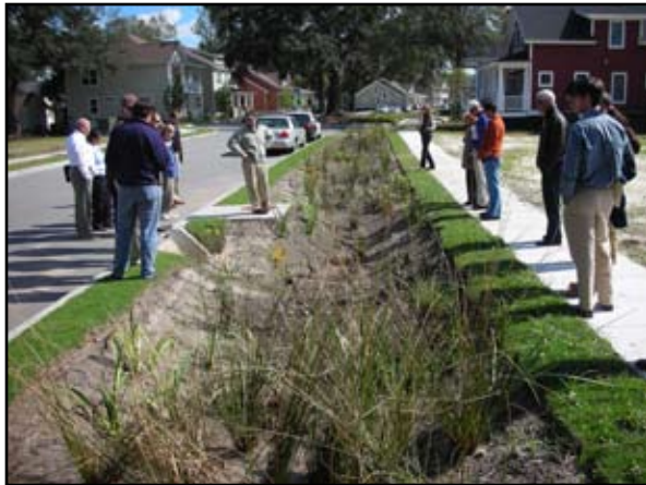
The Reserve partnered with SC Sea Grant to demonstrate bioswale installation and design at Oak Terrace Preserve, an innovative low impact development.
