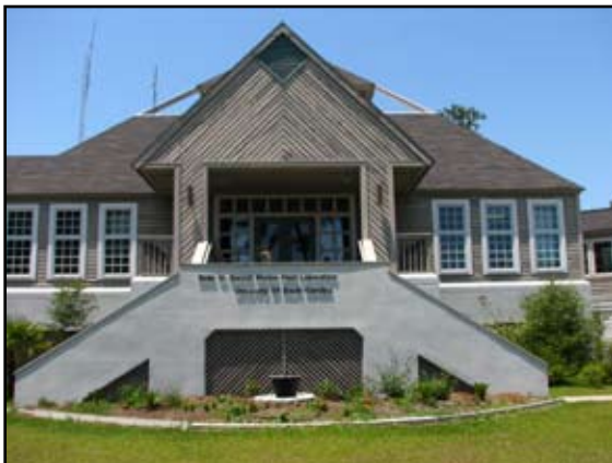
The Reserve would like to be able to retrofit some of the older facilities, such as the Baruch Marine Field Lab, with greener technologies and products.
