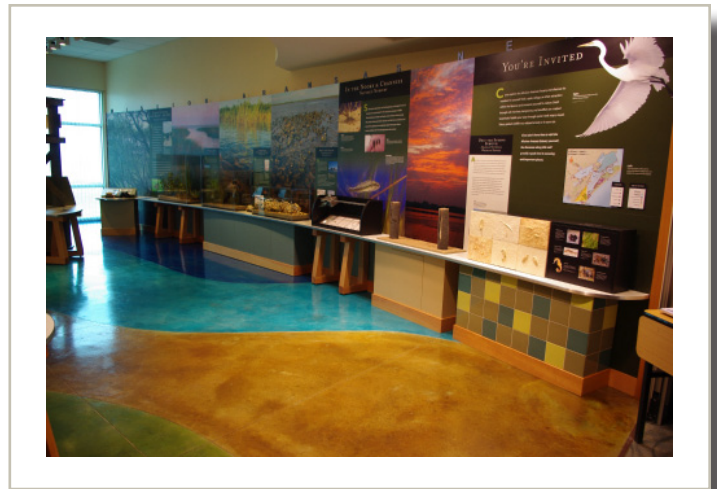
Painting of the concrete floors at the Bay Education Center improve aesthetics whiel also providing long-term durability
