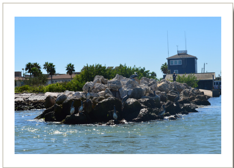
Rocks are used to create seawalls and breakwaters in the Mission-Aransas Reserve
