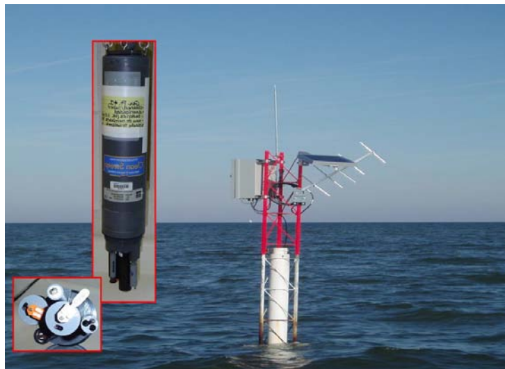
Figure 7.2. Goodwin Island SWMP continuous water quality monitoring station equipped with GOES satellite transmitter. Inserts: YSI EDS water quality datalogger. Photo credit: William Reay.
