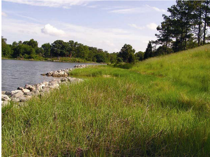
Figure 9.1. Example of a hybrid living shoreline erosion control structure. Photo credit: Karen Duhring.
