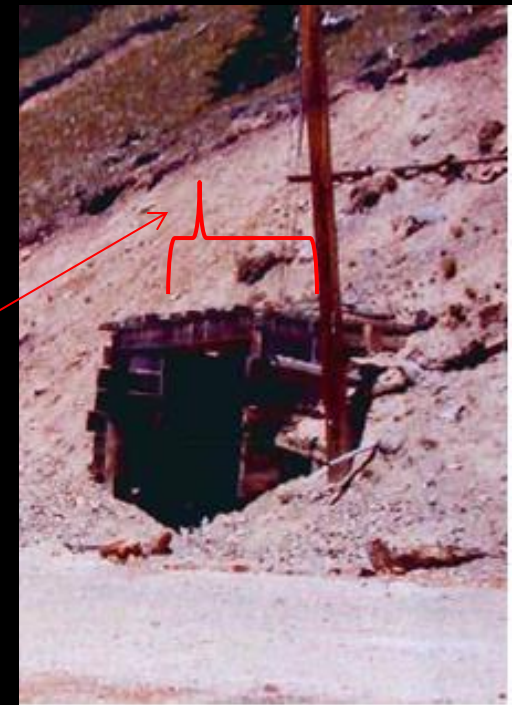
The adit in 2004. 2
