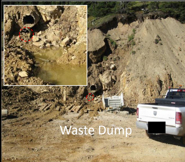
Drainage pipe (red) about level with waste rock dump in 2014. Inset: Pooling water.
