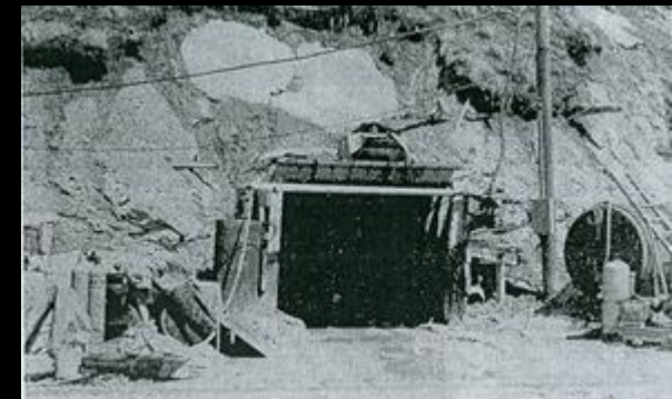
Portal Construction in 1984. 3
