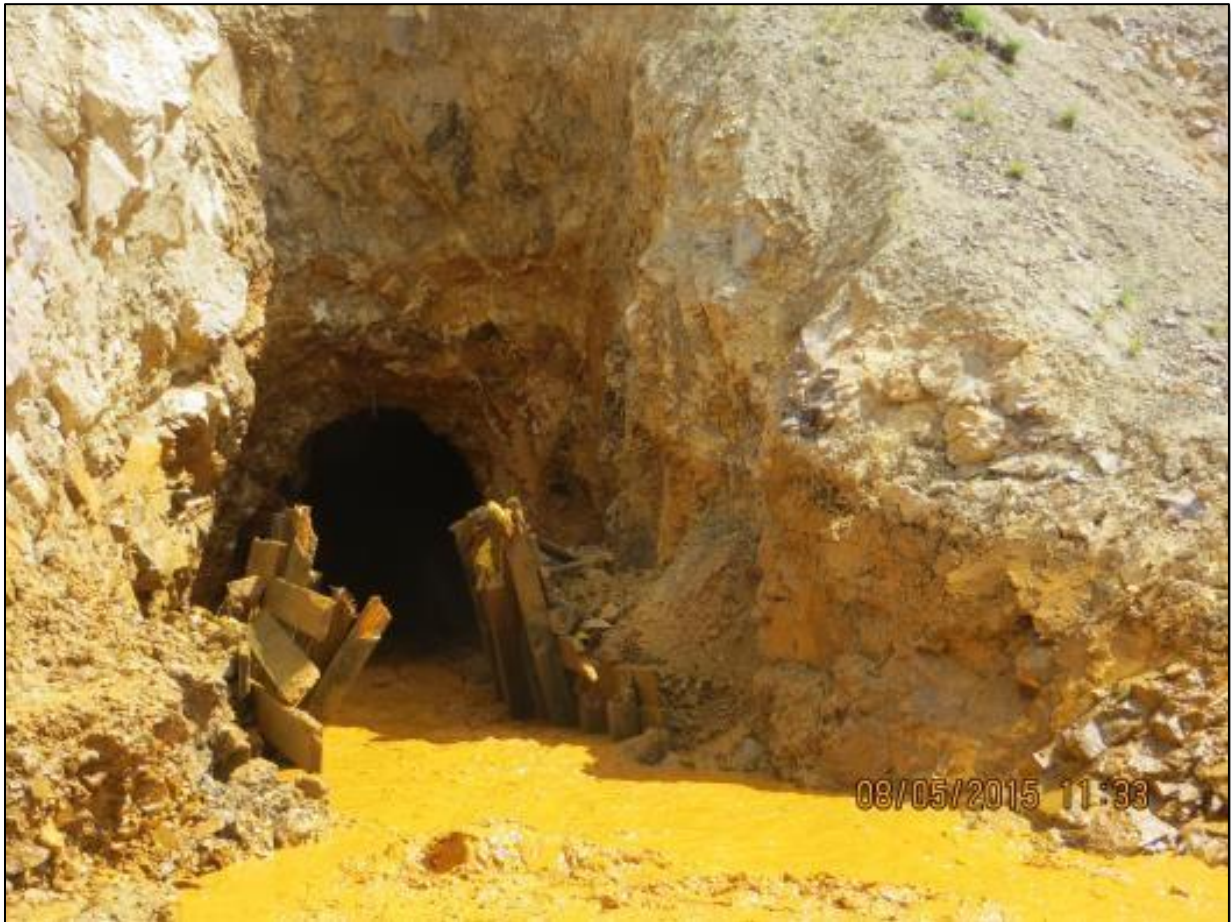
Entrance to Gold King Mine after EPA Caused the Blowout
