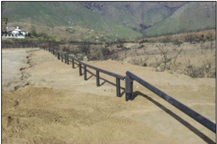
Figure 101b—Metal fencing to restrict vehicle access to an area that is naturally recovering.
