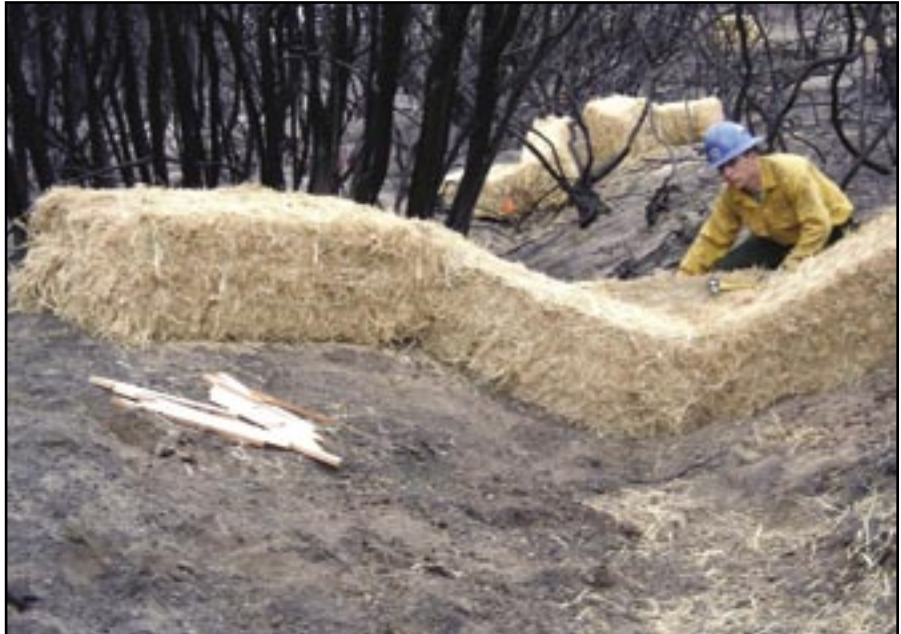
Figure 55—Install checkdams to avoid endruns.
