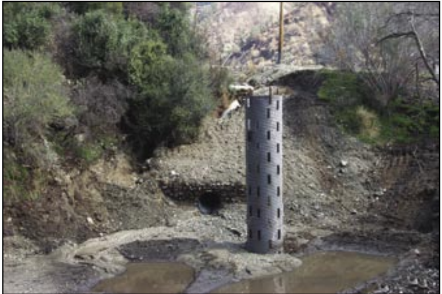
Figure 89—Tall riser used to prevent plugging of culvert.
