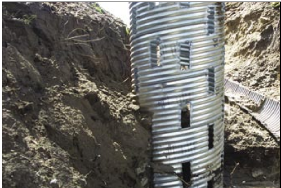
Figure 92—Ensure the openings on the riser are sized to allow water to flow freely into the structure. Small openings can plug with fine detritus.
