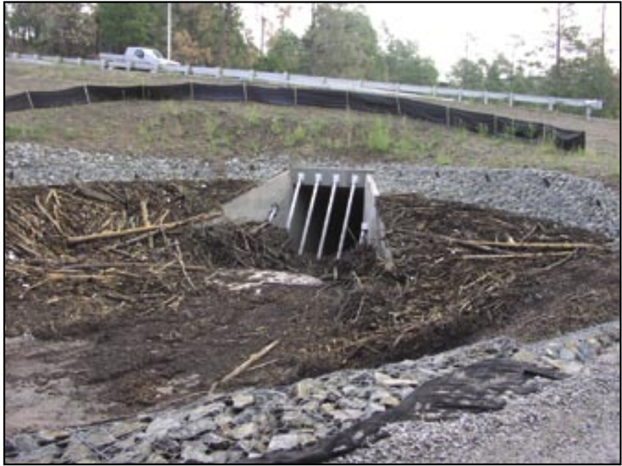
Figure 61—Ensure that material from the debris basin can be removed.
