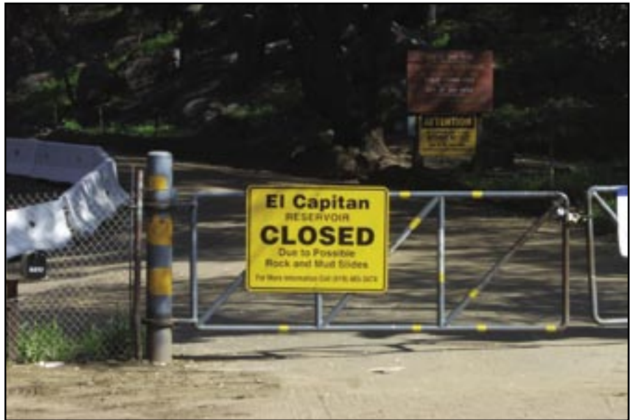
Figure 104—Gates prevent access to hazardous areas.
