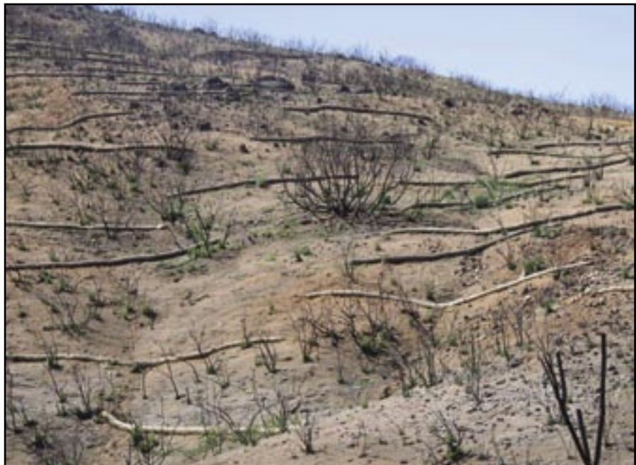
Figure 28—Fiber roll placed across the hillslope. Not all the fiber rolls are on the contour which can accelerate erosion.
