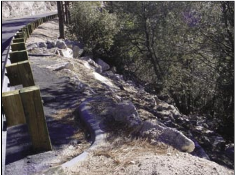
Figure 73—Imbricated rock level spreader is used on paved roads to protect the road fill.
