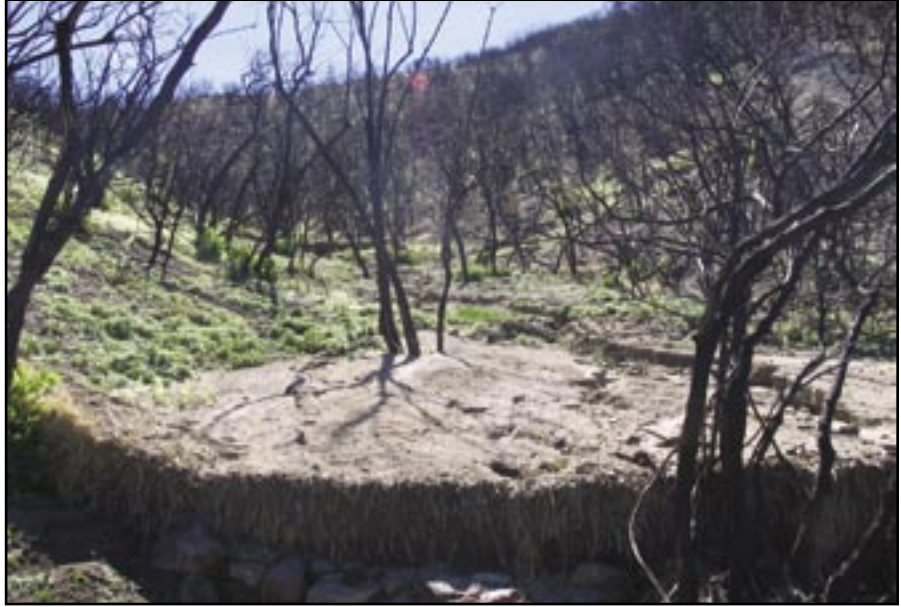
Figure 54—Checkdams should be inspected and maintained.
