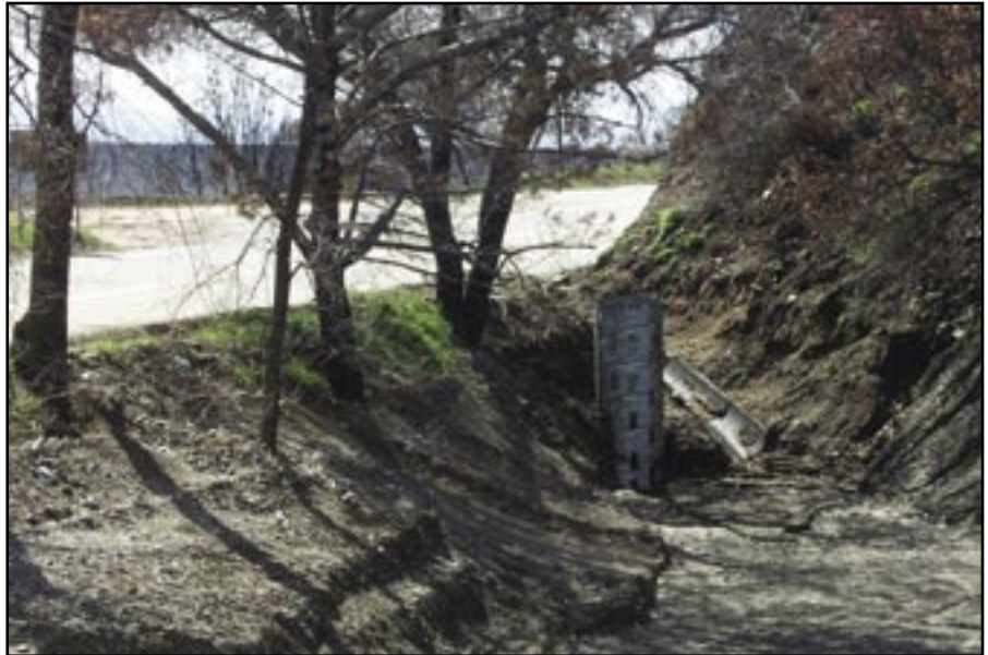
Figure 91—Riser located next to county road and receives frequent maintenance to remove material.
