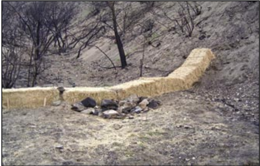
Figure 48—Strawbale checkdam with energy dissipater.
