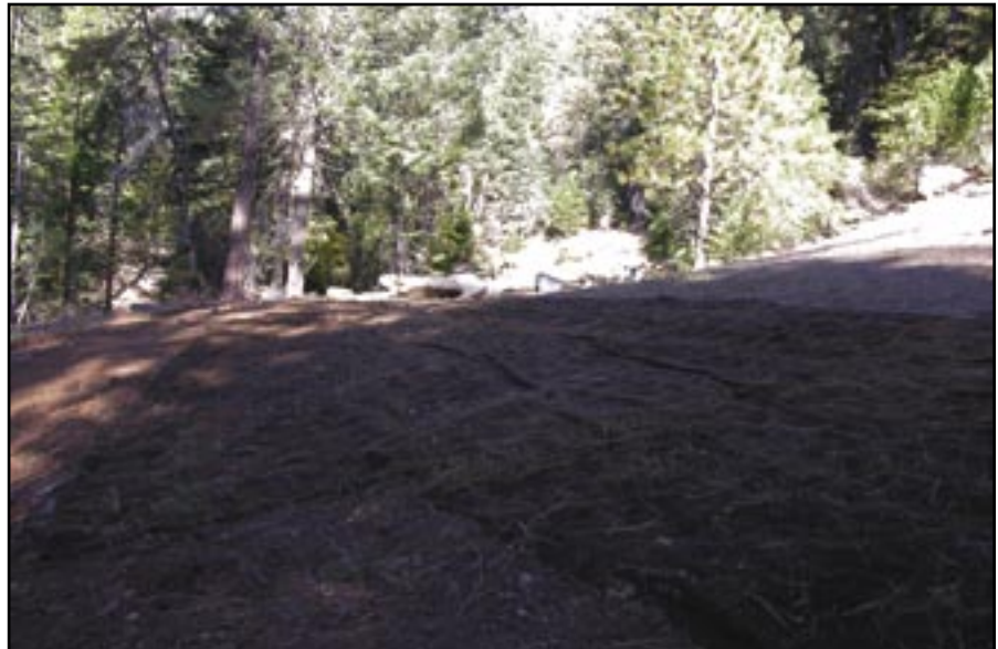
Figure 20—Proper implementation of erosion control mats ensures treatment success.
