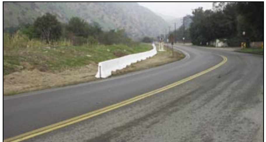
Figure 108—Jersey barriers can be removed from the road prism once the emergency is over.
