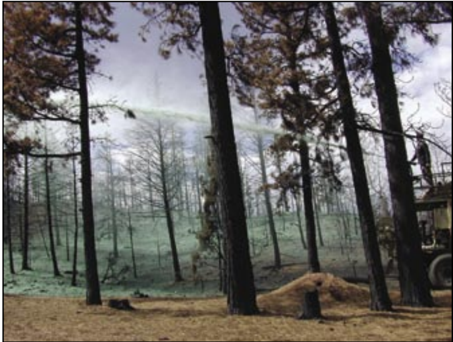
Figure 6—Ground application of hydromulch.
