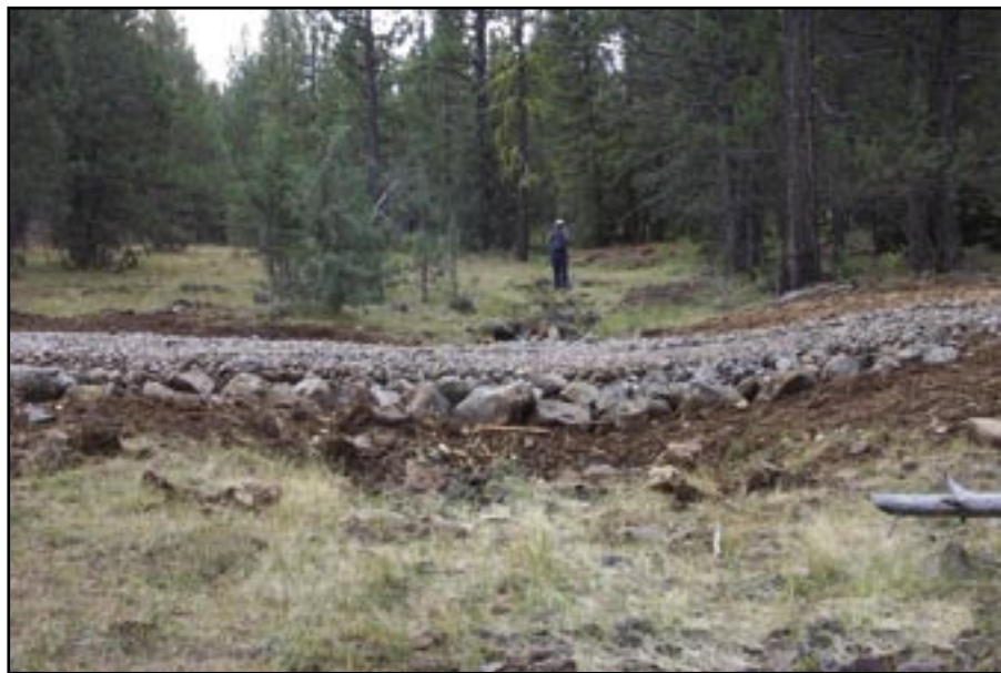
Figure 69a—Completed armored rolling dip.
