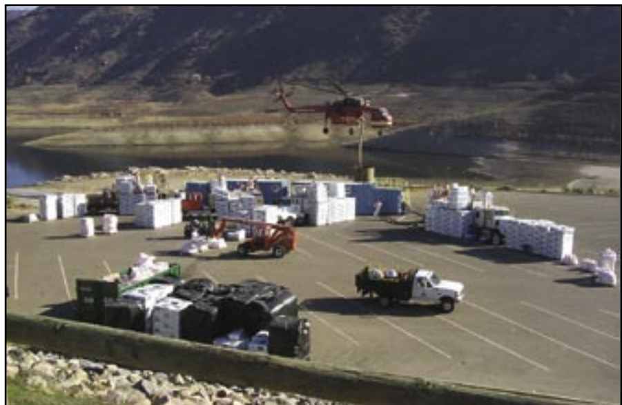
Figure 3—Aerial hydromulching requires close access to water, large staging areas, and close proximity to treatment units.
