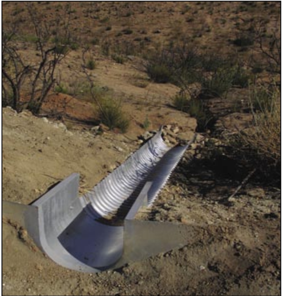
Figure 70—Metal roadside drain.
