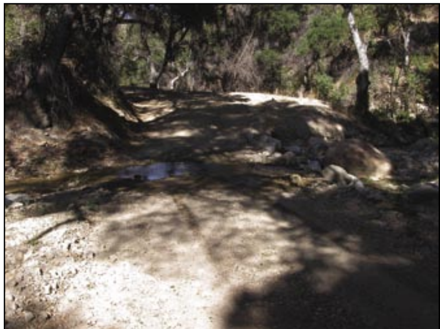
Figure 76—Low-water stream crossing replaces a 24-inch culvert.
