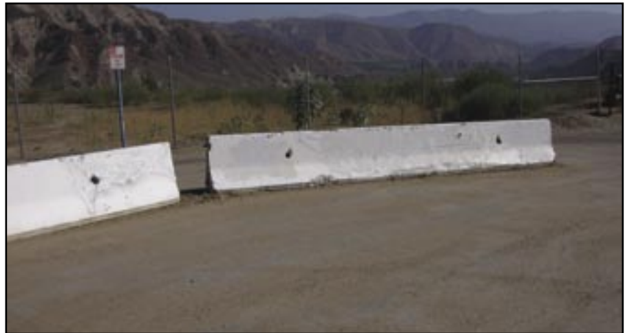
Figure 107—Jersey barriers (K-rail) can be used to limit vehicle access.
