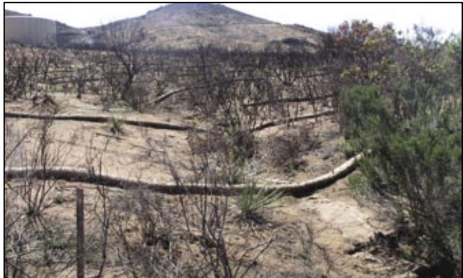
Figure 29—Avoid placing the fiber rolls in drainages.
