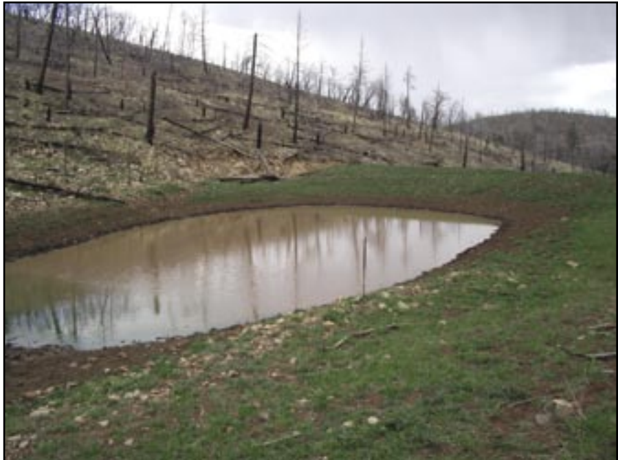
Figure 60—Small basin created to trap sediment.
