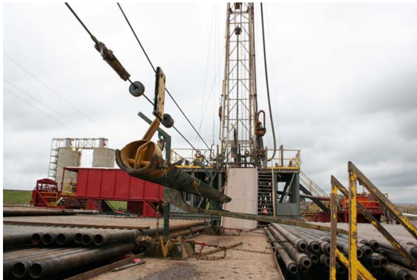
Figure 5-2 Typical drilling operations of a CO 2 injection well. Source: R. A. Esposito, Southern Company.
