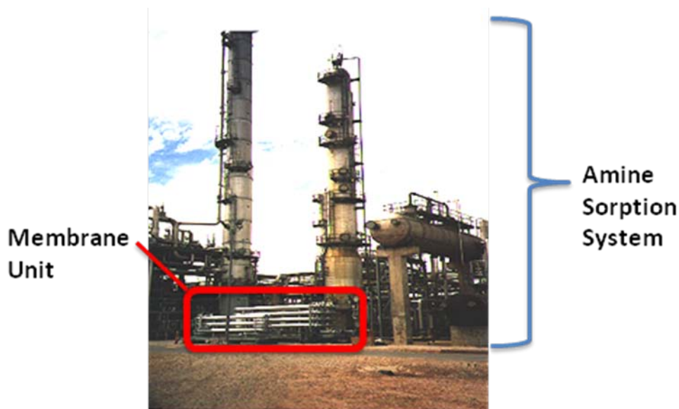
Figure 6. Comparison of a membrane unit with a conventional separation process (i.e., amine absorption system) for removing CO 2 from natural gas. This figure shows the mechanical simplicity of membrane systems as well as their space efficiency relative to other separation processes. Courtesy of Air Liquide.
