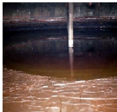
Figure 1: At the Hanford site, 53 million gallons of high-level radioactive and chemical waste are stored in 177 underground tanks.
