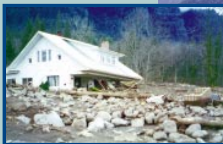
This debris flow occurred in the Columbia River gorge near the town of Dodson, Oregon, during a rainfall and snowmelt event in February 1996 (Photo Inset: S. Cannon, USGS). The combination of rainfall and snowmelt resulted in severe flooding and landsliding throughout the Pacific Northwest. The debris flow shown here was deposited in a number of separate events over a period of 2 days. The flows originated high on the palisade and traveled through the steep canyon. The occupants of the house escaped with their lives when they heard a loud rumbling and crashing of trees and saw the approaching material through their kitchen window. Boulders, mud, and debris from these and several nearby debris flows were deposited across the east-bound lanes of Interstate Highway 84, and blocked the highway for 5 days (Aerial Photo: D. Wieprecht, USGS).
