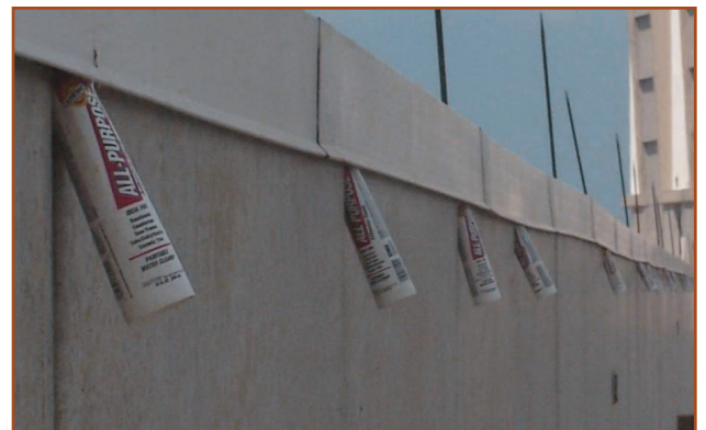
Figure 12. In long areas, place eviction tubes about 6 feet apart along the entire distance to enable all the bats to exit. (Source: Fly By Night Inc.)
