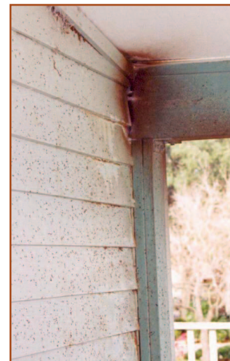
Figure 10. Staining can indicate a bat entry/exit point. (Source: Fly By Night Inc.)
