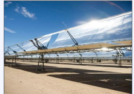
Concentrated Solar Power
