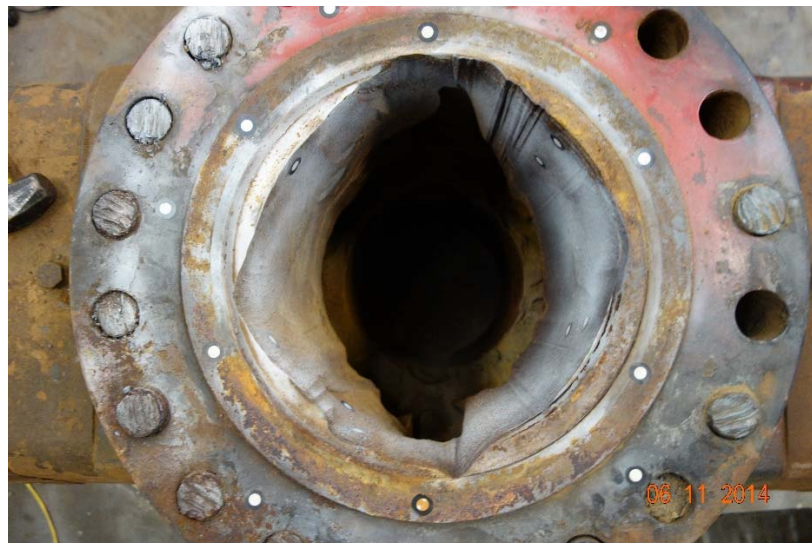
Figure 8.2 – Photograph looking down through bore of Lower Ram Body
