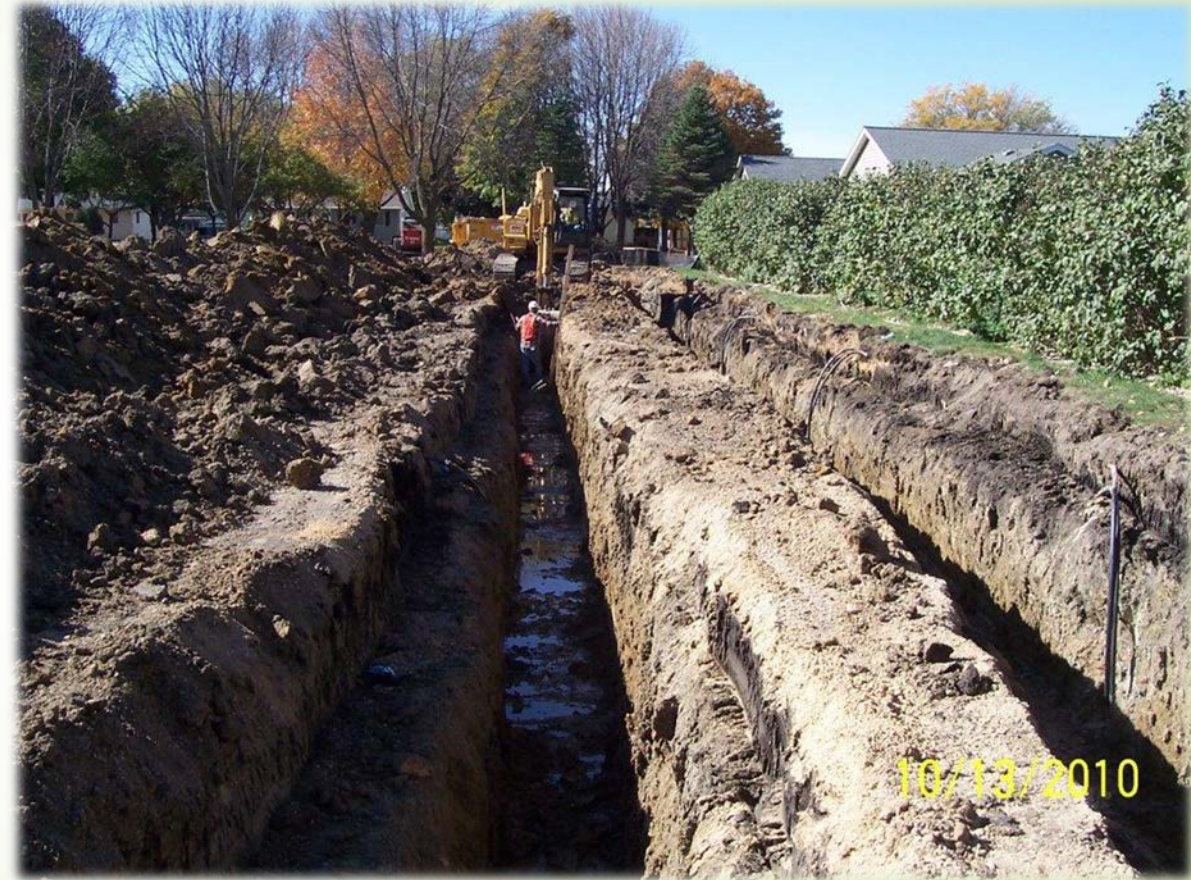
Digging Geothermal Wells
