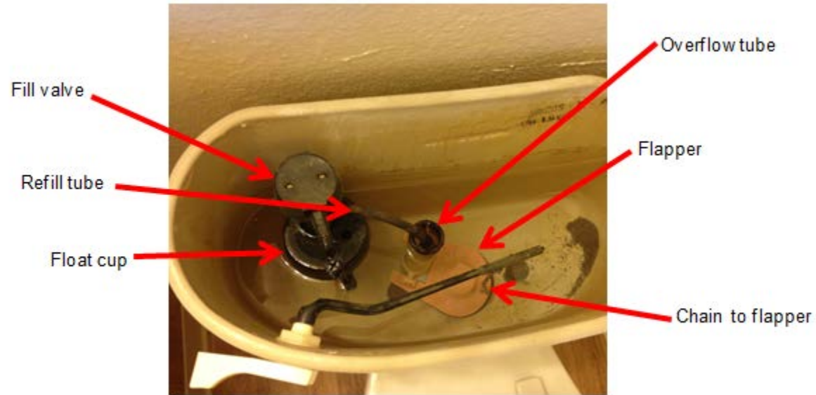
Figure 24 - Toilet Components
