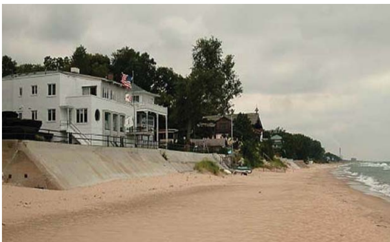
Figure 3-8 Shoreline Protection Structure, 2004 – Near Michigan City, IN on Lake Michigan
