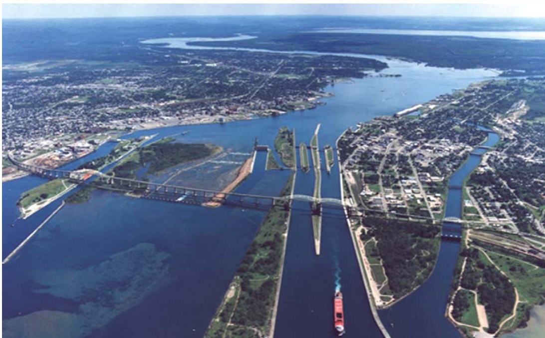
Figure 11-1 Lake Superior Regulation Control Structures
