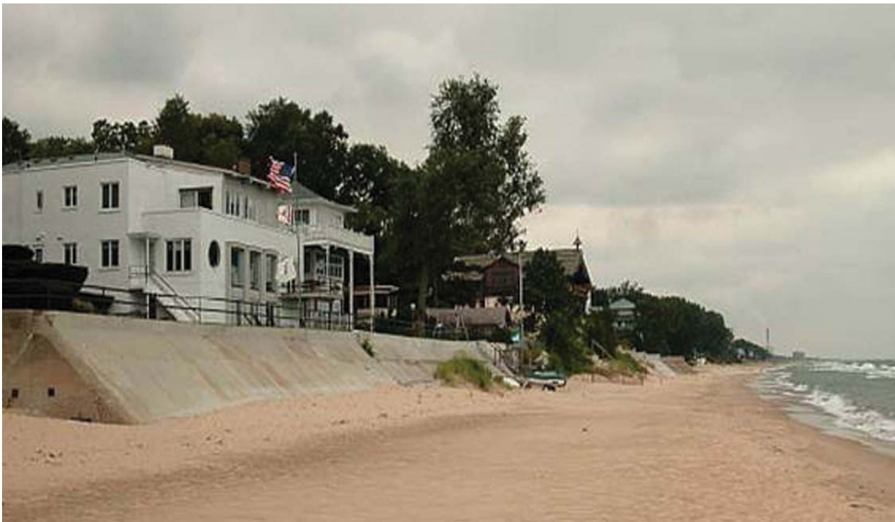
Figure 11-4 Shoreline Protection Structure, 2004 – Near Michigan City, IN on Lake Michigan
