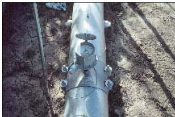
Figure 1. Flow meter for closed pipe.
