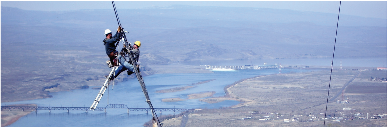
BPA linemen install a helical connector shunt on the Midway-Vantage 230-kV line in central Washington, north of Hanford.
