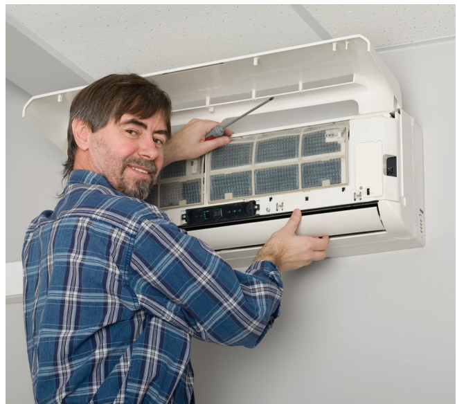
Ductless heat pump systems use 30 to 50 percent less energy to heat homes than electric-resistance or forced-air systems.
