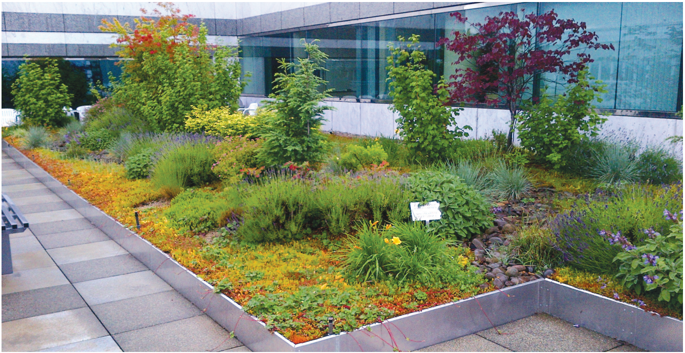
BPA's eco-roofs reduce stormwater by capturing and evaporating an average of 60 percent of the rain that falls on them.
