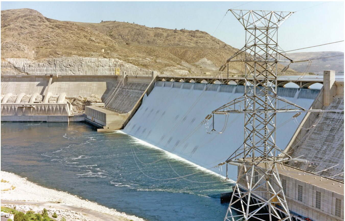
Grand Coulee Dam
