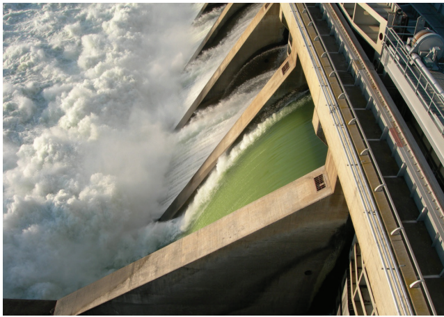
The smooth green flow of spill over a surface passage route provides a safer way for young fish to migrate downstream.
