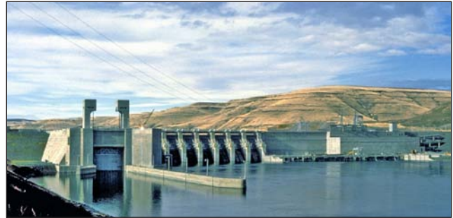
Ice Harbor Dam — capacity 603 MW, energized 1961
