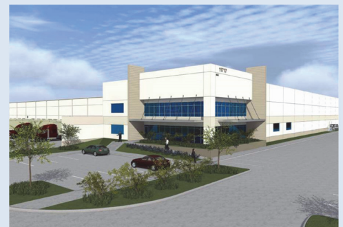
Lennox International's leased regional distribution center in Houston, Texas. Photo courtesy of Lennox International.
