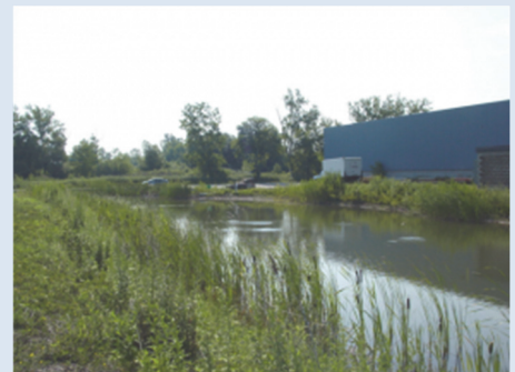
A view of HARBEC’s 1.2 million gallon-capacity water-retention pond. Photo courtesy of HARBEC.
