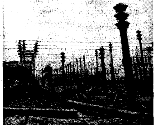
Construction of the Ross Substation about 1938. Those are mules or horses being used !
